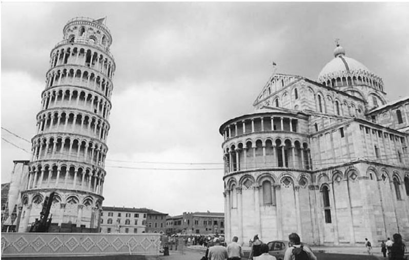
Figure 6.4 The Leaning Tower, Pisa, Italy. Photo by Michael Calia, copyright 2003. Permission to publish requested by the author and granted by the photographer.
