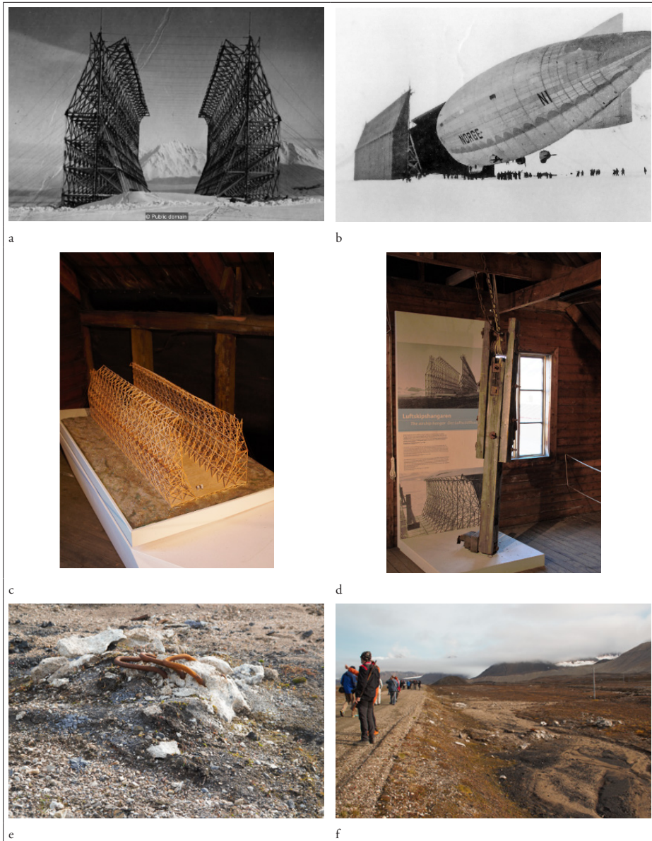
Fig. 86 – Historical pictures and current remnants of the polar airship base at Kings Bay; a) the hangar before application of sailcloth covers; b) NORGE being pulled into the hangar; c) scale model of the hangar; d) surviving element of the hangar; e) element of the hangar structure in situ; f) traces of hangar structures along the road
