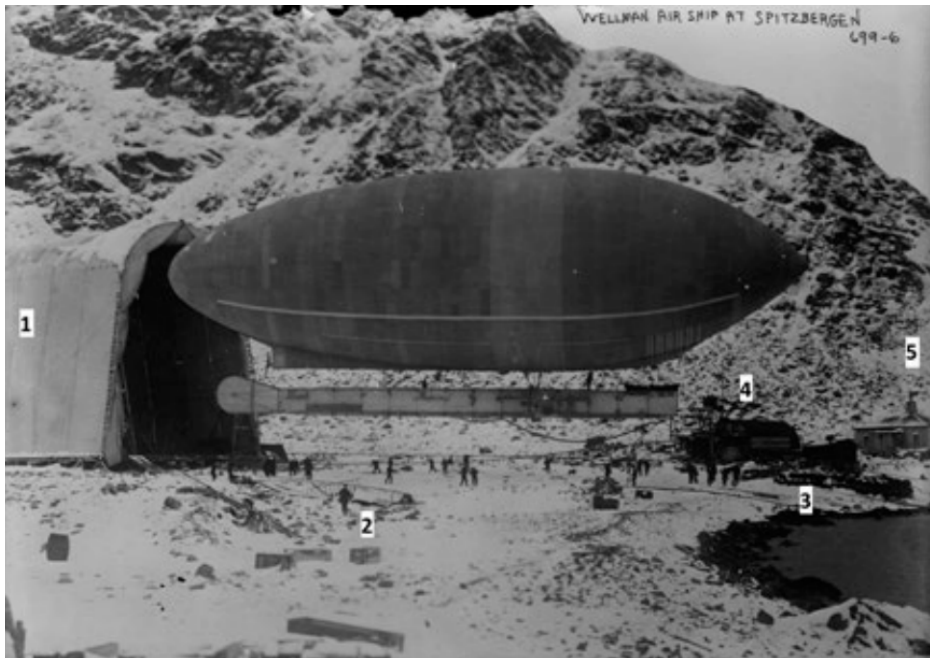
Fig. 104 – Airship AMERICA at Virgohamna just outside of the hangar (1), in 1907. In the foreground, an object laying on the snow next to a standing person could possibly be the structure – after removal of the fabric cover – of the first airship gondola, built by Godard for the 1906 expedition (2). On the right, it is possible to see the large stack of fuel barrels (3). Technical buildings are visible in the background (4) and so is Wellman's Hut (5). Over a century after this image, even very lightweight and mobile objects were still visible approximately in the same locations. This is evident by comparison with figure 105
