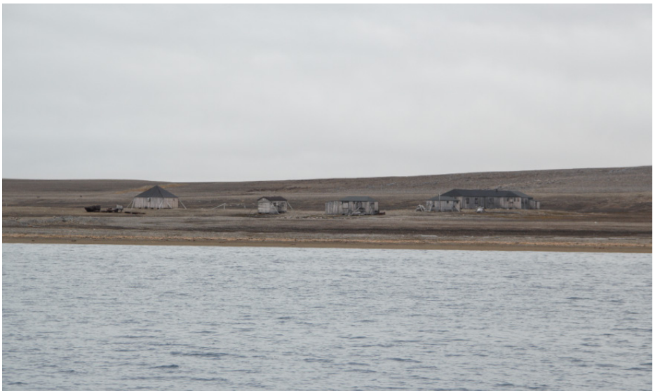
Fig. 57 – Buildings in the central area of Kinnvika station
