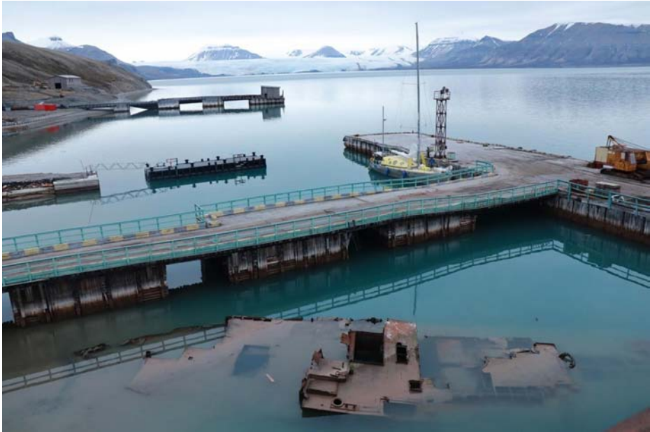
Fig. 81 – Pyramiden harbour appeared fitted with minimal equipment and services to allow for small to medium boat/ship activity. Much of the Soviet day infrastructure for larger ship traffic was in an evident state of decay. In the foreground, the wreck of a sunken boat surfaces from the shallow waters; Nordenskjöldbreen is visible in the background
