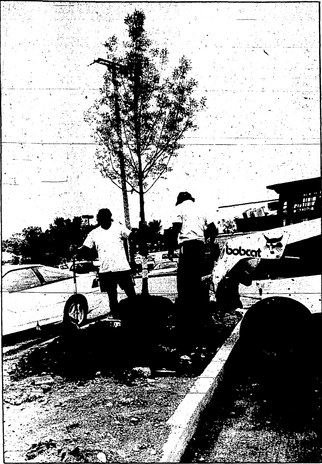
Bank deposit? Landscape company employees place a large tree in the Comerica Bank parking lot Monday, the bank's first day of lobby business after several months of renovation and expansion.
