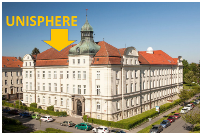
Fig. 1 Unisphere is located in attic space of this building.
