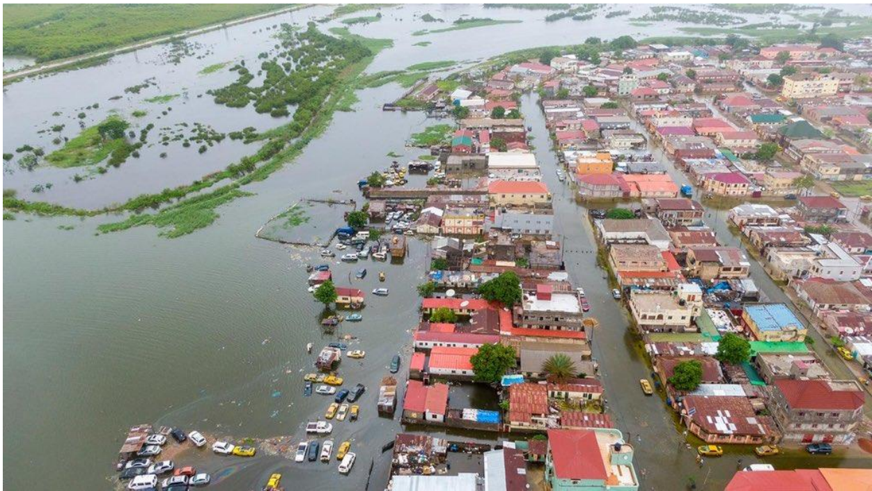
Figure 2 Photograph depicting the 2022 flooding of Tobacco Road neighborhood in Banjul. The green vegetation in the top left of the image are mangroves, which prior to the reclamation of this
