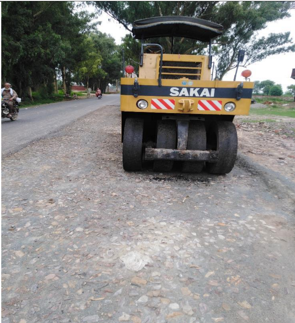
Figure 10: Deployment of Construction Machinery at the site
