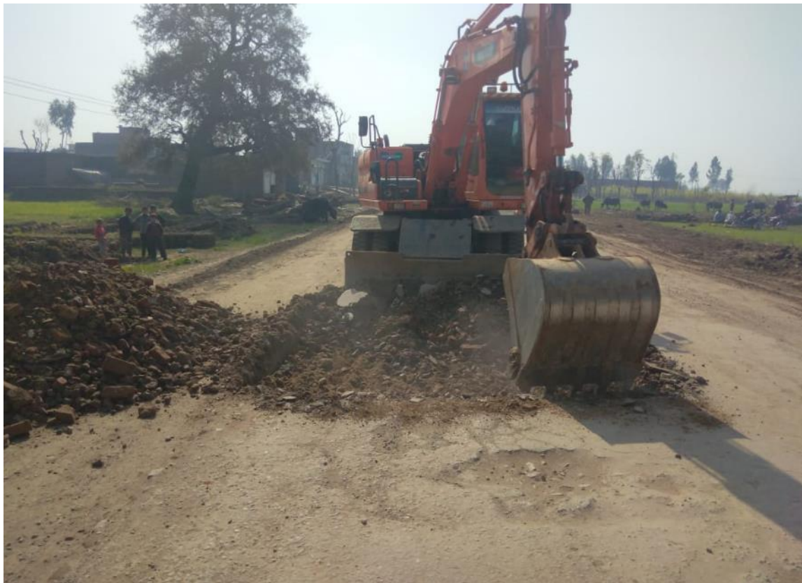
Figure 6: Work in Progress on the road
