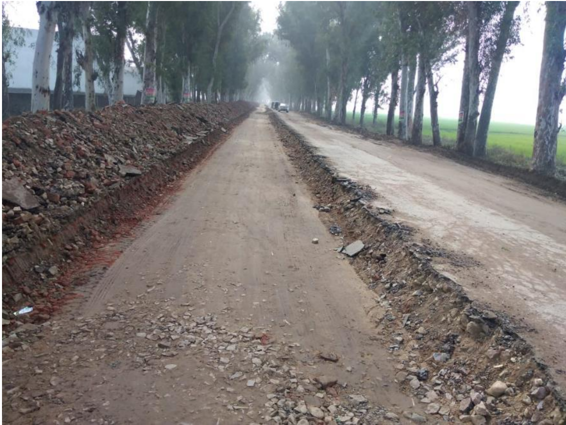
Figure 5: Excavated Road for Compaction purposes
