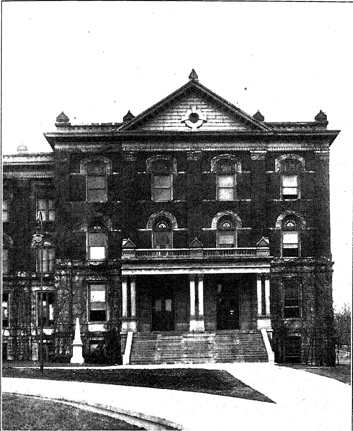
WEST WING JESSE HALL Where the Library was Housed 1895 to 1915
