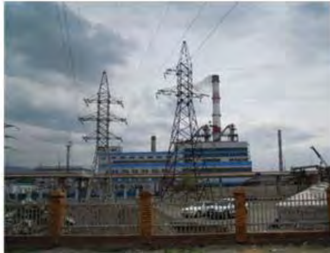
Fig. 4-2 Full View of Power Plant, Chimney: 120m (The 80m-chimney at left is not used)
