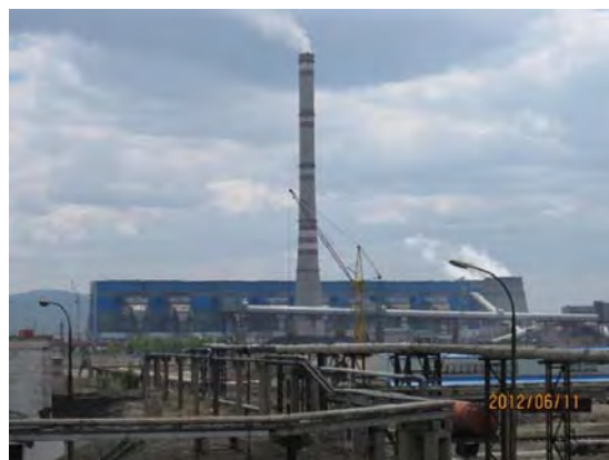
Fig. 4-8 Full View of Fourth Power Plant from Boiler Building Side (Picture taken from second power plant, pipes in the foreground are for factory steam)
