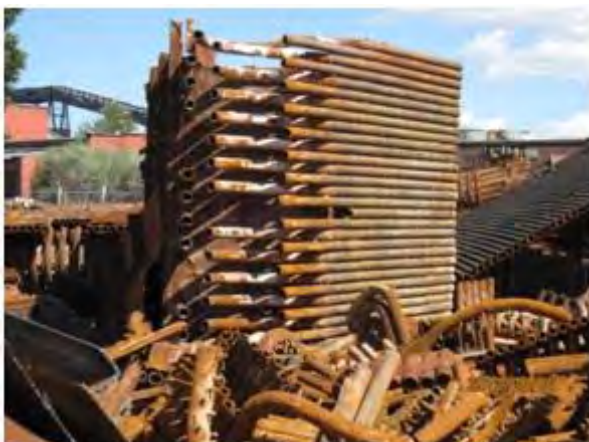
#13 boiler: 100% tube relocated Tubes dismantled and located outdoor
