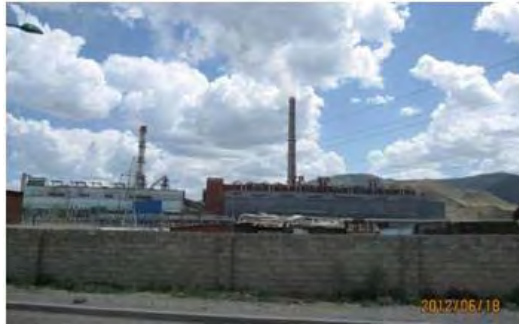
Fig. 4-4 Full View of Power Plant
