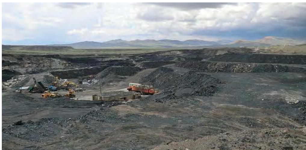
Fig. 3-16 Panoramic View of Mining Pit in Khotgor Coal Mine
