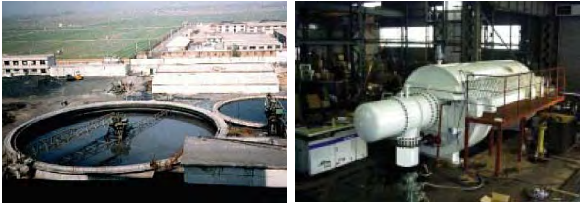
Fig. 5-10 Thickener (right) and dewatering device (left)
