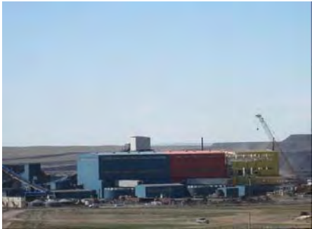
Fig. 3-7 Coal Preparation Plant
