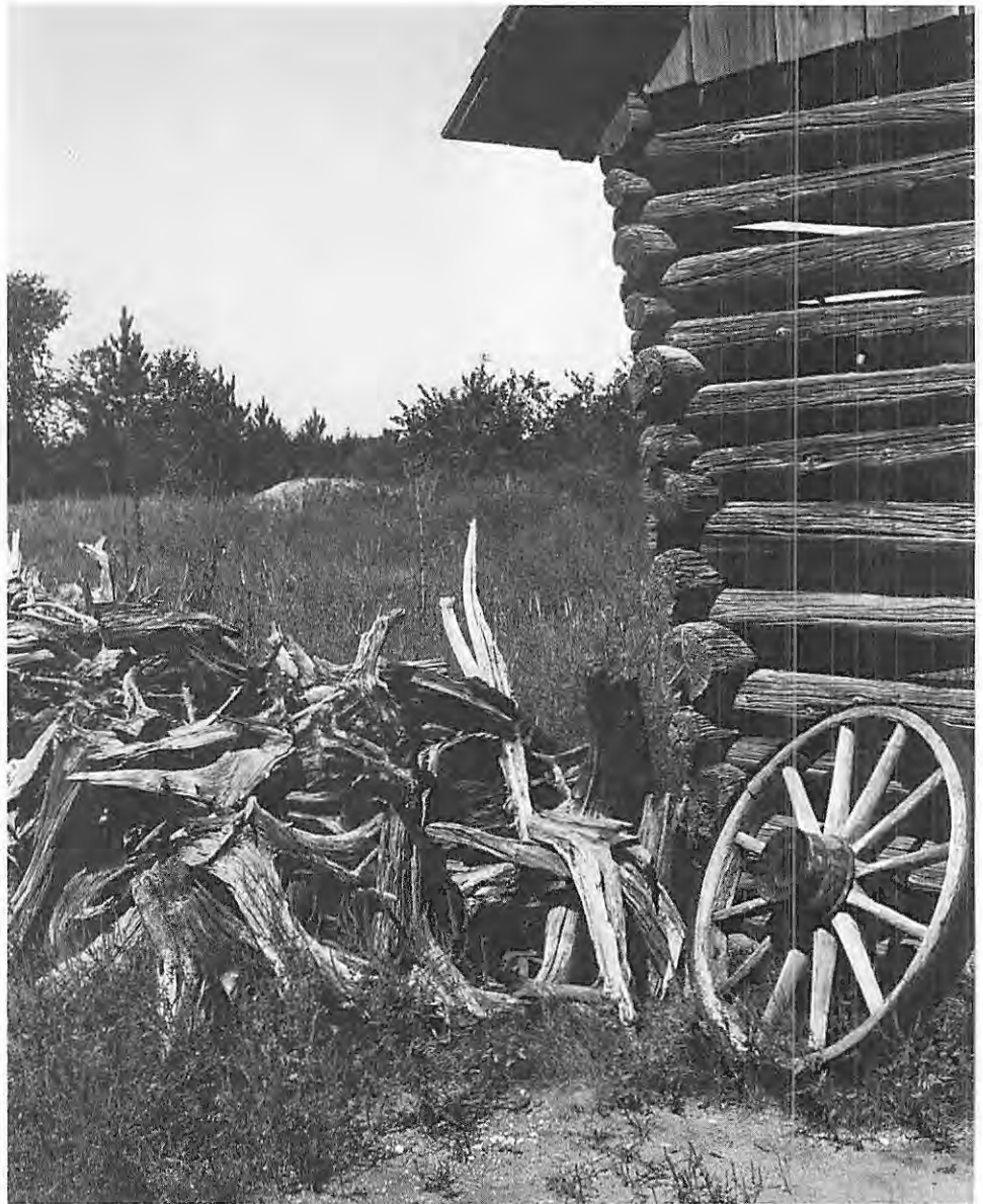
Stump fence and Lantta Hay barn in the Finnish area at Old World Wisconsin. The Finnish farmstead complex, among the most well developed, preserves the rural architecture of one of Wisconsin's later (1880s–1920) arriving immigrant groups in rich detail. The barn was built with loose fitting logs to allow ventilation and slanted walls to promote rain runoff. The Finns farmed in the cutover lands of Douglas, Iron, and Bayfield Counties, Wisconsin. The Finns laboriously pulled stumps left by the lumbermen, often using them for fences such as the one pictured here. Photo by Margaret Bogue.
