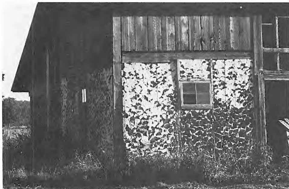
Stovewood log barn located about 4 miles northwest of Baileys Harbor on County Trunk F. Photo by Margaret Bogue.
