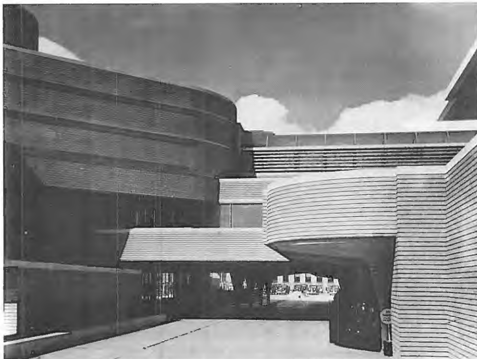
The S. C. Johnson and Sons, Inc., office building, designed by Frank Lloyd Wright, about 1948. Courtesy State Historical Society of Wisconsin. WHi(X3)54
