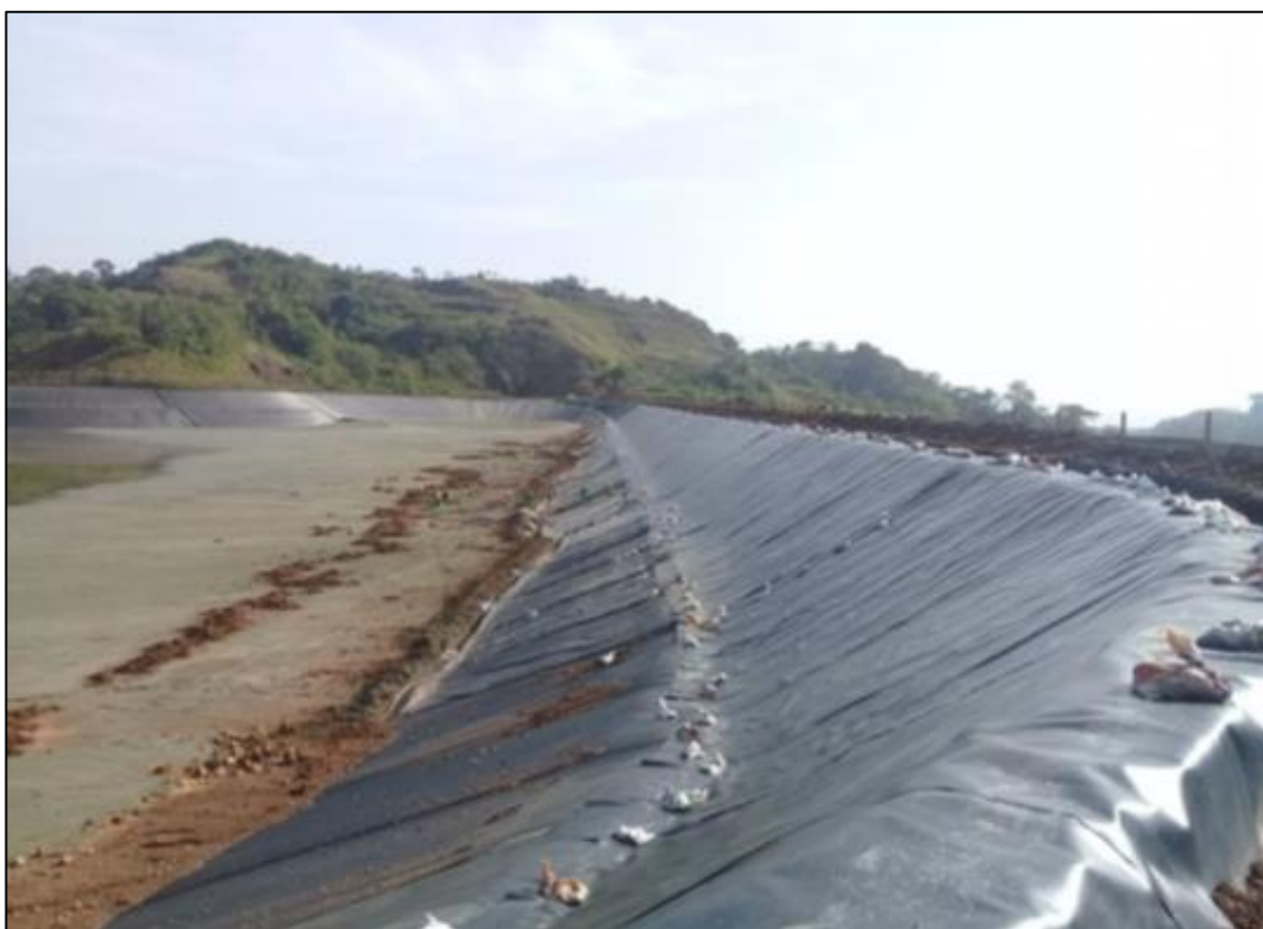
Figure 17.18 – La Soledad Dam Raising and Lining
