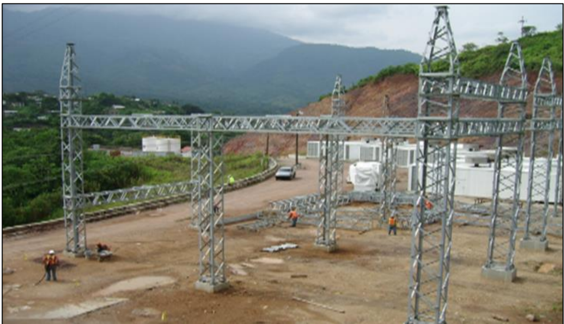
Figure 18.7 – 69 kV substation under constructions
