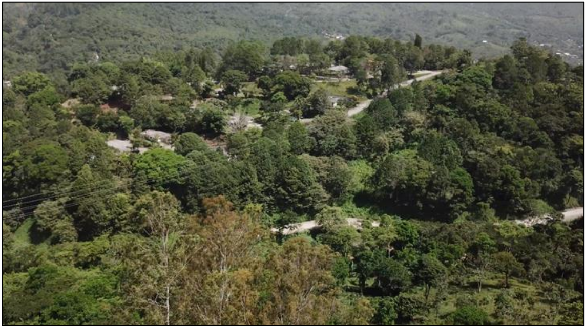
Figure 18.13 – Aerial view of the mine village
