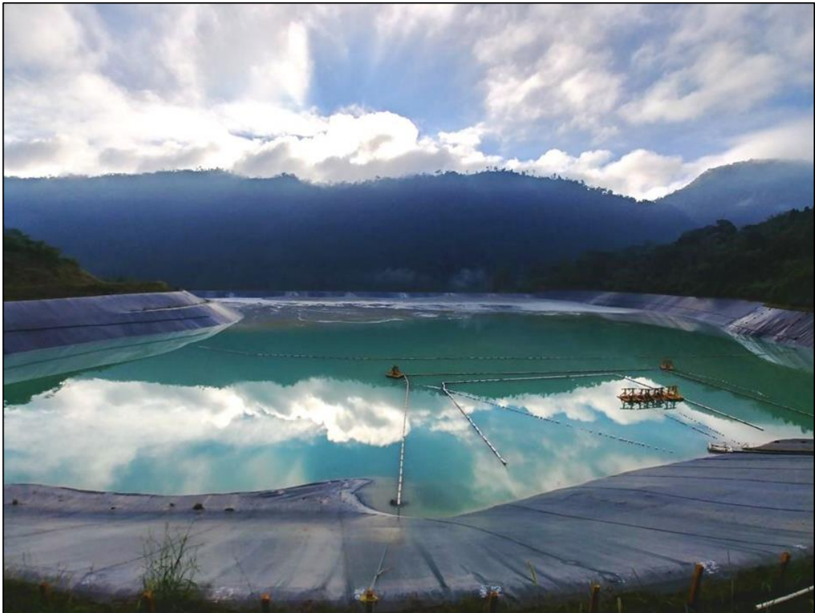
Figure 18.17 – Soledad TSF and Stage 4 wall lift, looking East
