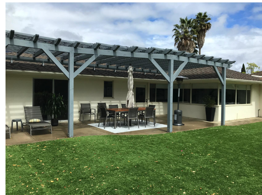
BACKYARD 36 LA FLECHA LN (FROM BACK RIGHT)
