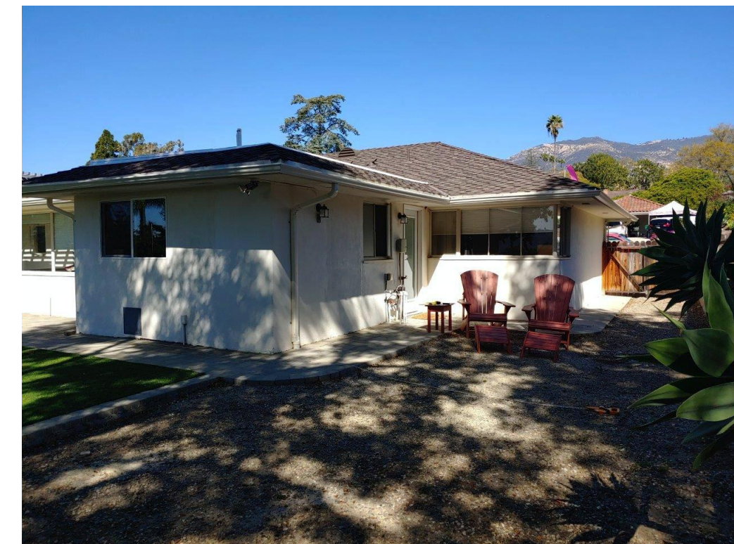
BACK OF 36 LA FLECHA LANE (LEFT)
