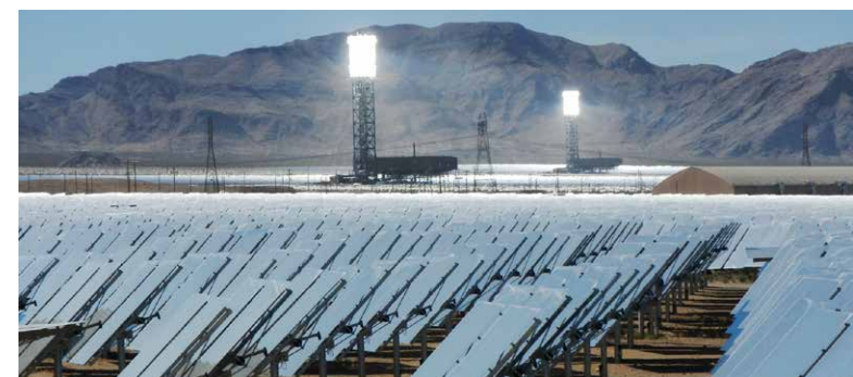
The Ivanpah Solar Electric Generating System is an example of a concentrated solar power plant, which works by having hundreds of reflective panels heating up a central tower. The problem of keeping sunlight directed at the receiver throughout the day brought Jim Clair to request NASA's help in validating the suspended design now used in Skysun solar power systems. Credit: Cliff Ho/U.S. Department of Energy
