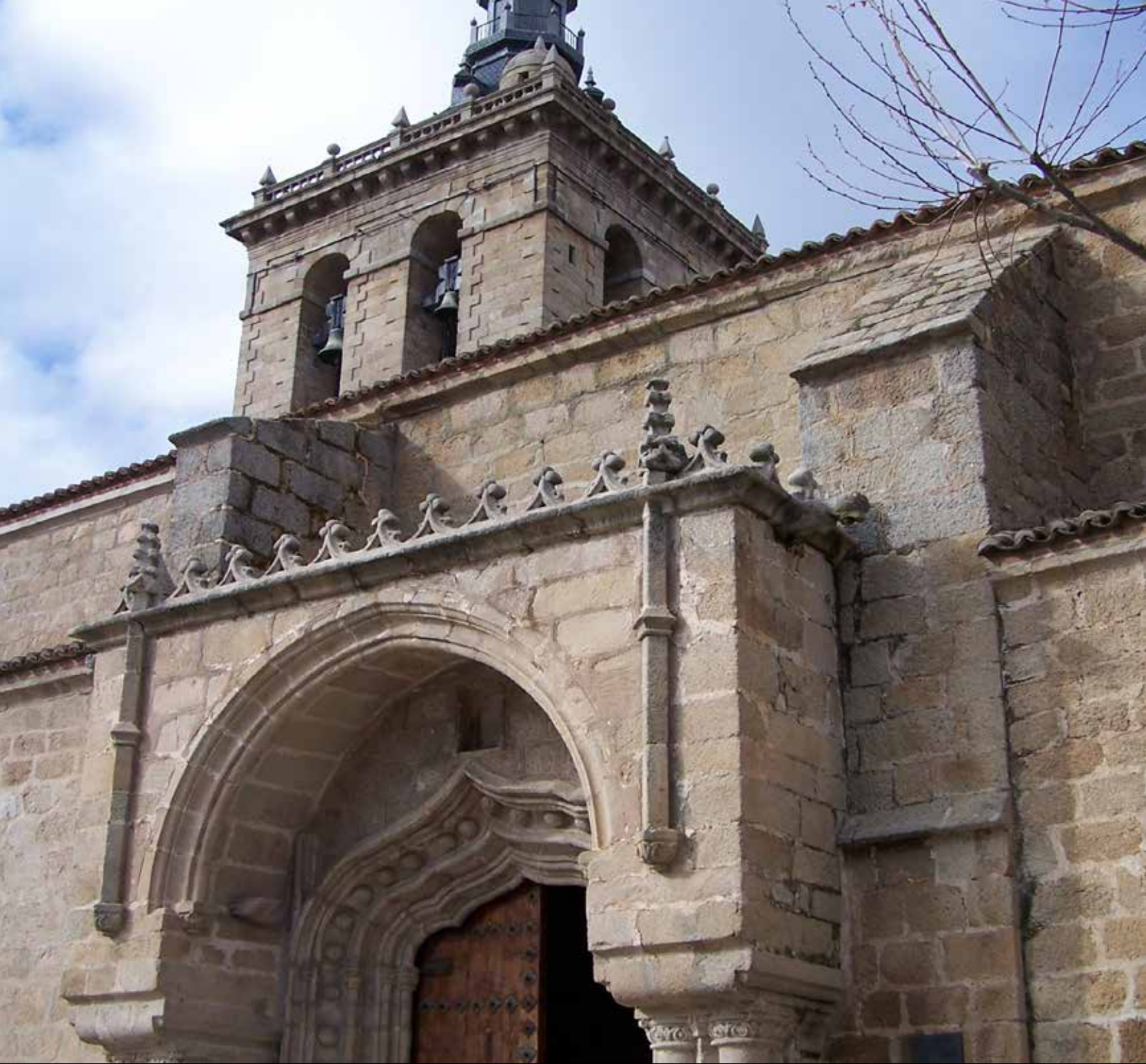
IGLESIA DE SANTIAGO APÓSTOL / CHURCH OF APOSTLE SANTIAGO
