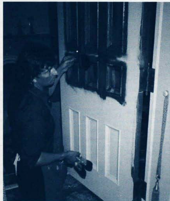
Above: The exterior restoration included replacement of the front windows. Below: An artisan grains the parlor doors to resemble cherry wood.
