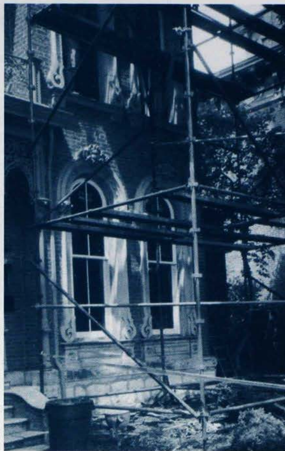
Above: The exterior restoration included replacement of the front windows. Below: An artisan grains the parlor doors to resemble cherry wood.
