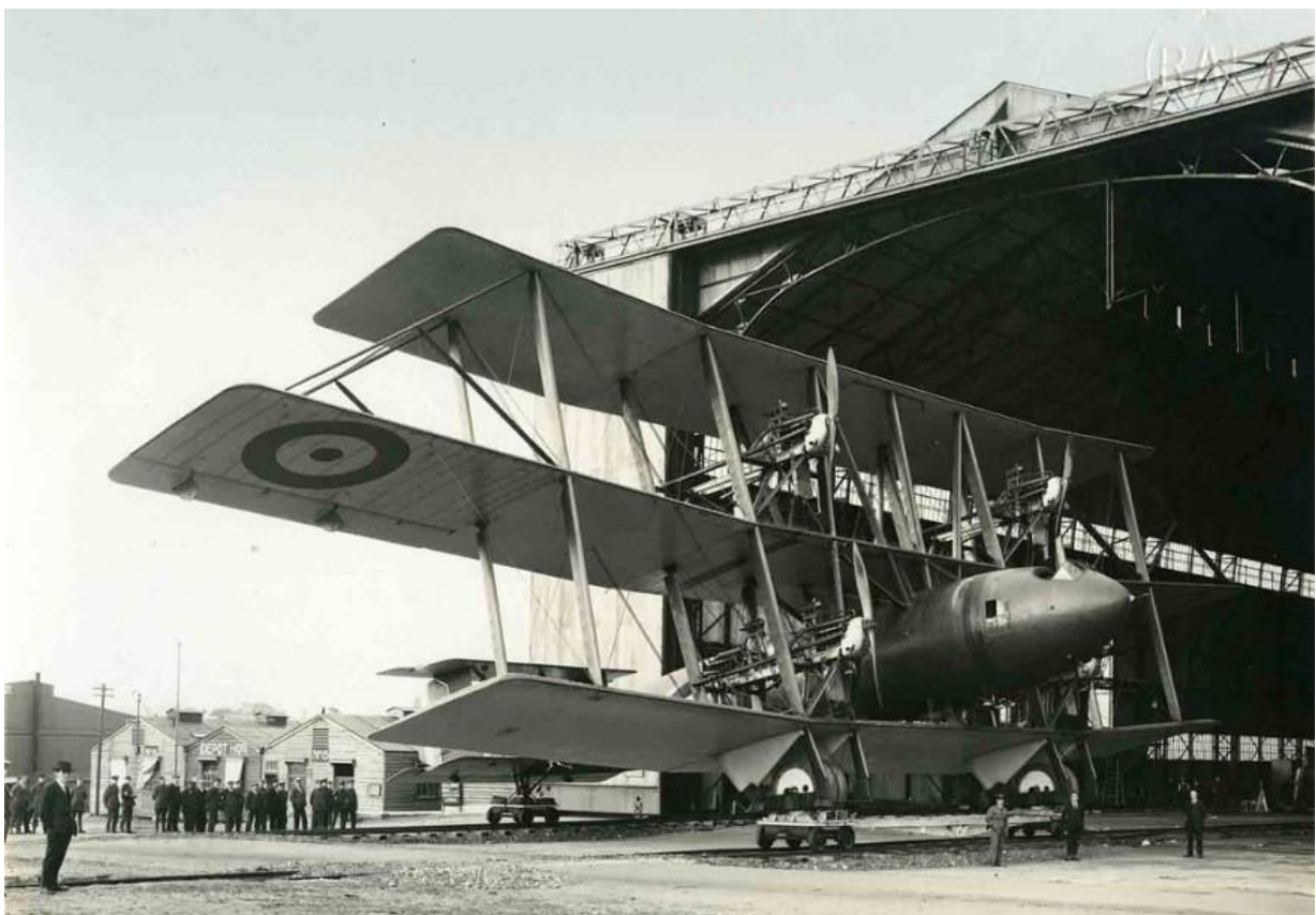
Figure 29. The Tabor on its track outside the gigantic ‘C’ Shed. The rails sank below the wide dirt road, allowing the machine to be winched forward onto solid ground.
