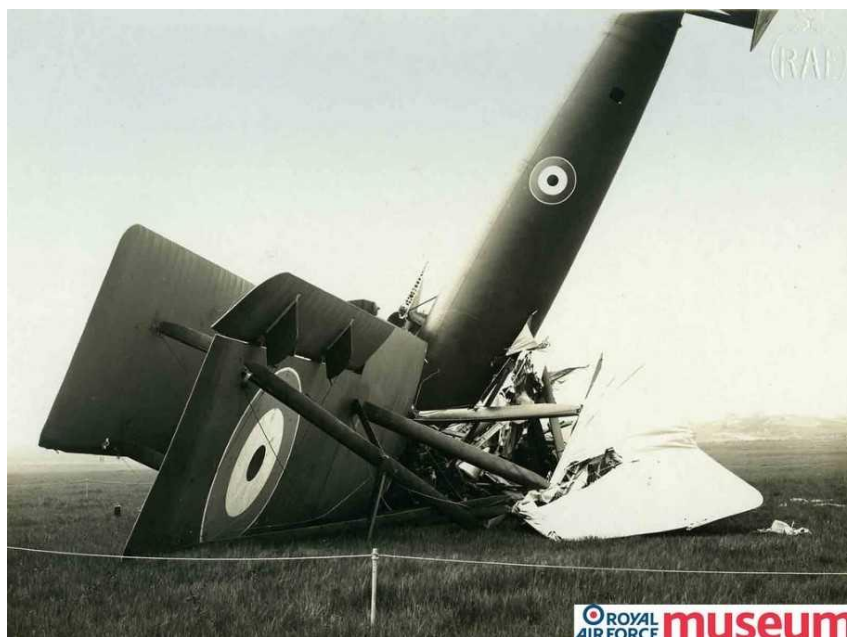
Figure 41. The Tabor from the starboard side, showing total destruction of the nose and top wing.
