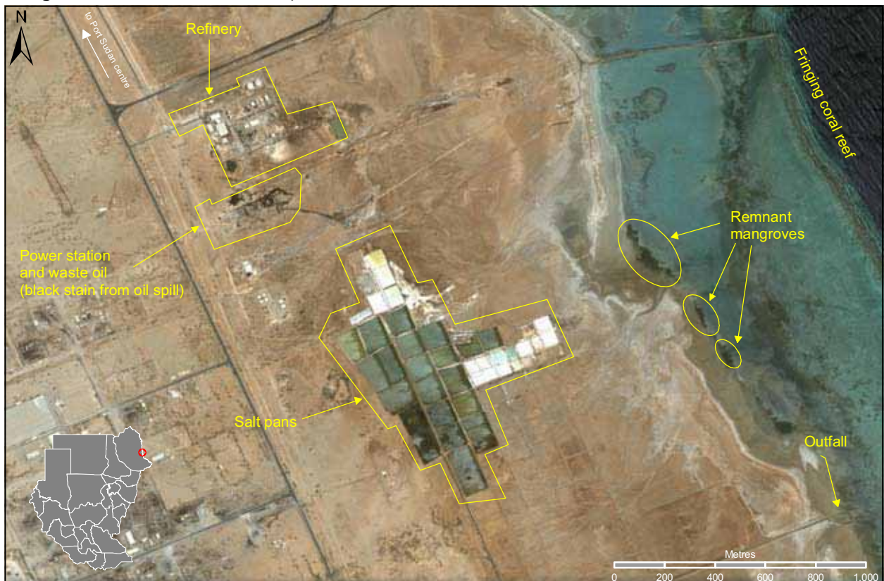
Figure 12.3 Port Sudan power station and salt flats
