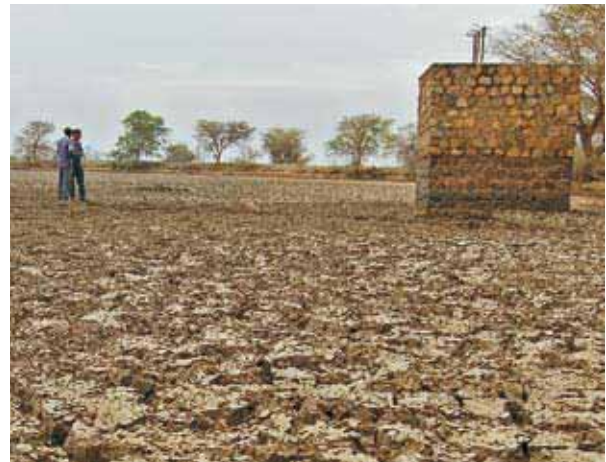
Lack of investment and maintenance during the conflict years led to complete or partial loss of many hafirs, such as this one at El Tooj, near Talodi in Southern Kordofan. Constructed in 1972 as part of a national campaign to eradicate thirst, the water treatment facility was targeted during the conflict and local communities have been drinking untreated water ever since
