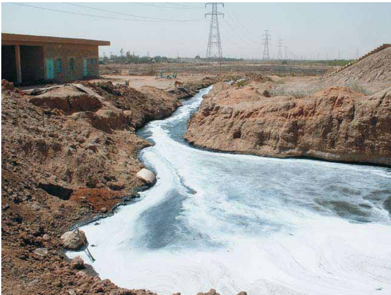
Raw sewage flowing to the White Nile. Though there is a sewage network in Khartoum, it does not cover the entire city and no longer works properly, as it is stretched well beyond capacity
