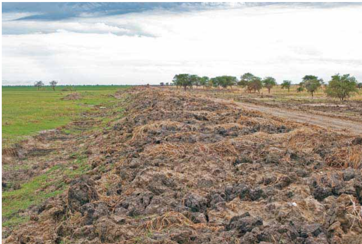
The dyke by the Bor-Padak rural trunk road was dug to control flooding in the region, but is now a cause for concern as it is leading the land beyond it to dry out and is thus reducing grazing land for both livestock and wildlife
