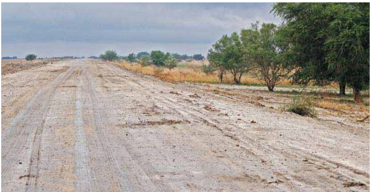
The unfinished Juba-Malakal trunk road project includes a 250 km stretch to be built on the west bank of the Jonglei canal. Approximately 100 km had been built by mid-2006, opening this remote area up for development
