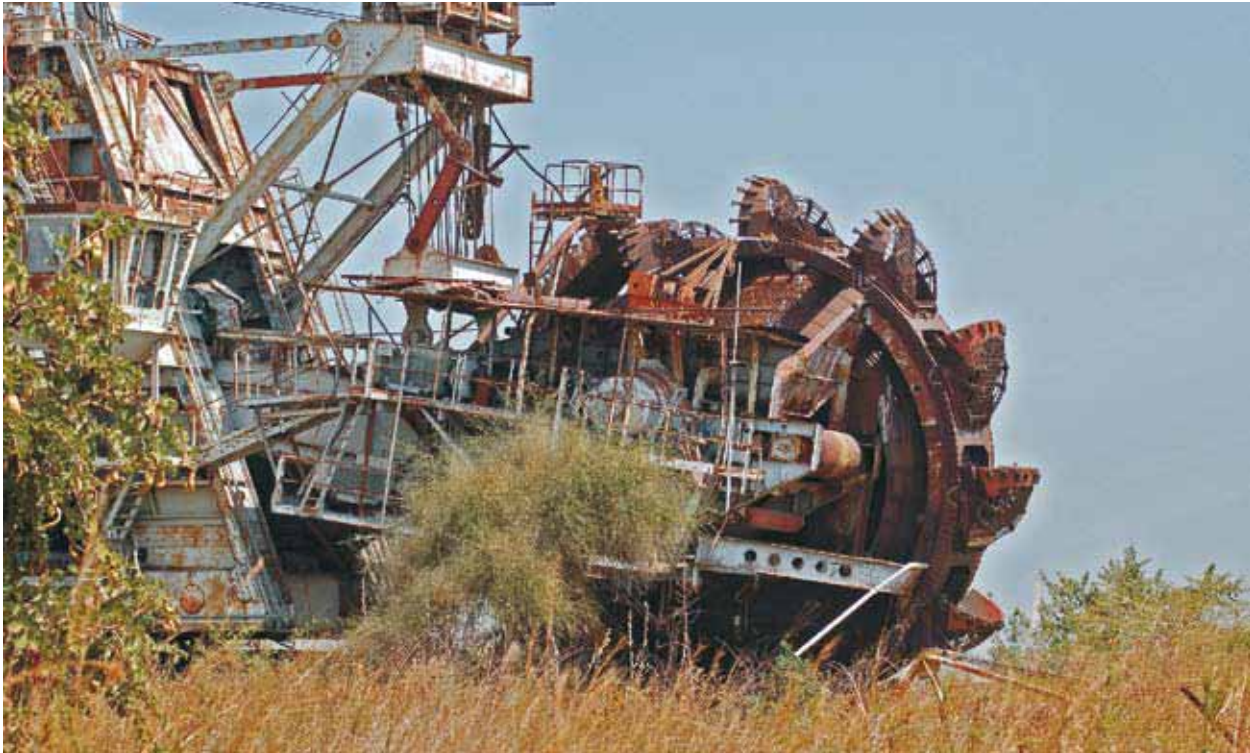
The rusting wreckage of the Jonglei canal excavator lies in the unfinished main channel. This failed venture illustrates the risks associated with developing large-scale projects in socially and environmentally sensitive areas without local support
