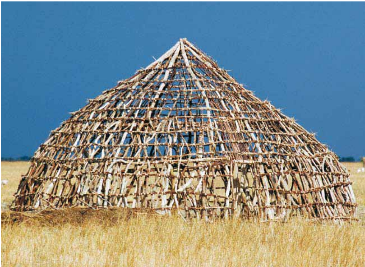
Traditional buildings such as this barn under construction near Mabor in Jonglei state require a large number of young trees
