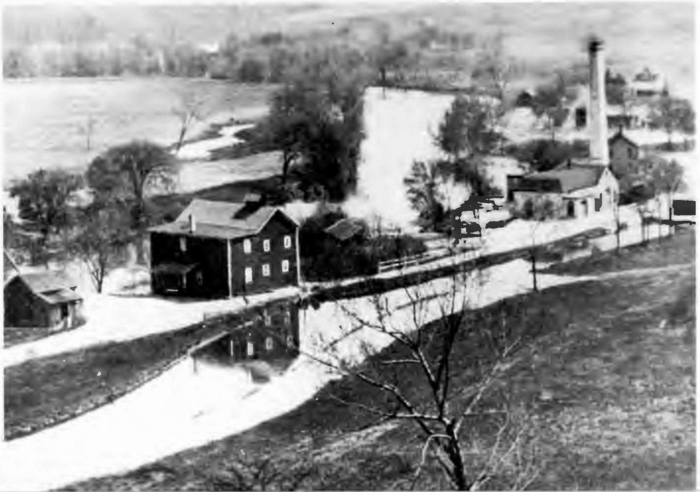
City Water Pumping Station
