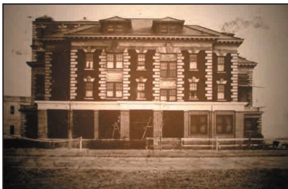
Figure 17: Nurse's Home west elevation, alterations in 1937 by the WPA. Source: The New York Public Library Local History Division.
