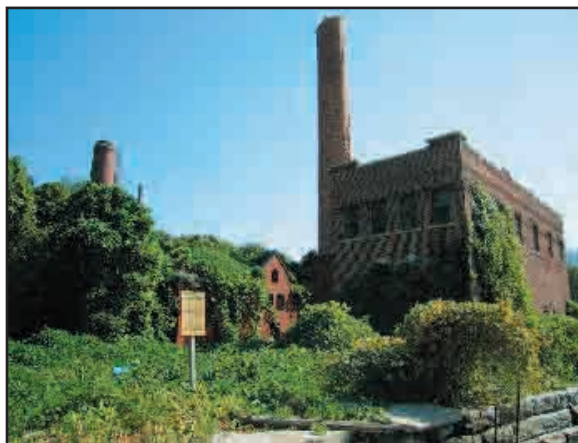
Figure 3: Boiler room (left) and Morgue (right), note extensive kudzu growth, view southeast (Hillary Adam, 2005)
