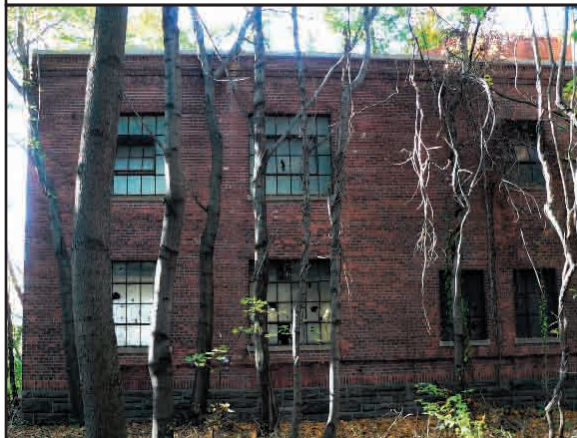
Figure 18: Shop and Storage Building. (Kelly Wong, 2005)
