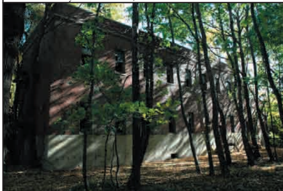
Figure 14: West elevation of 1929 Service Building. (Kelly Wong, 2005)
