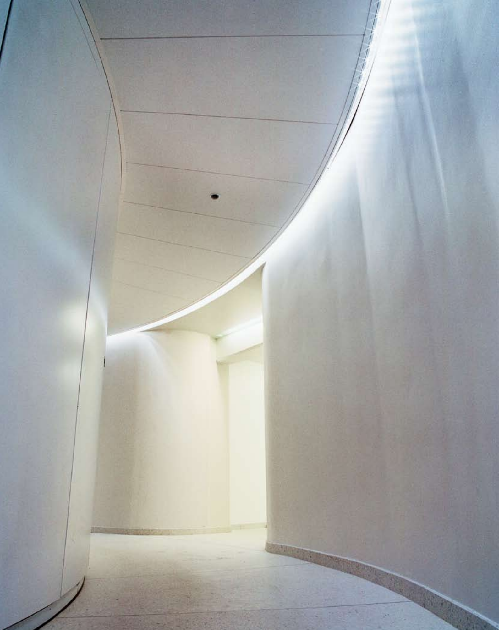
The design of the Turning Torso means that the corridors are circular. Consequently, the fixtures used in the corridors need to follow the same curve. Conventional fluorescent lamps would have thrown uneven lighting on the walls, whereas LED lighting creates an even lighting.
