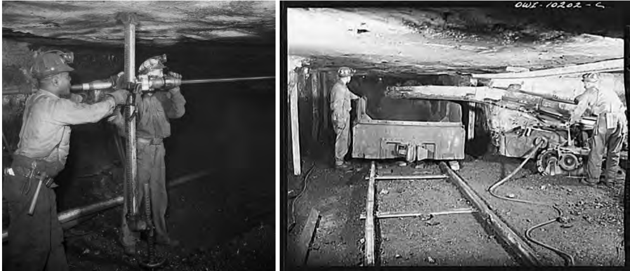
Pittsburgh Coal Company, Montour no. 4 mine (L) Drilling, (R) Mechanical loader filling mine car, Pittsburgh, PA vicinity, 1942 (John Collier, LOC P&P, FSA/OWI)
