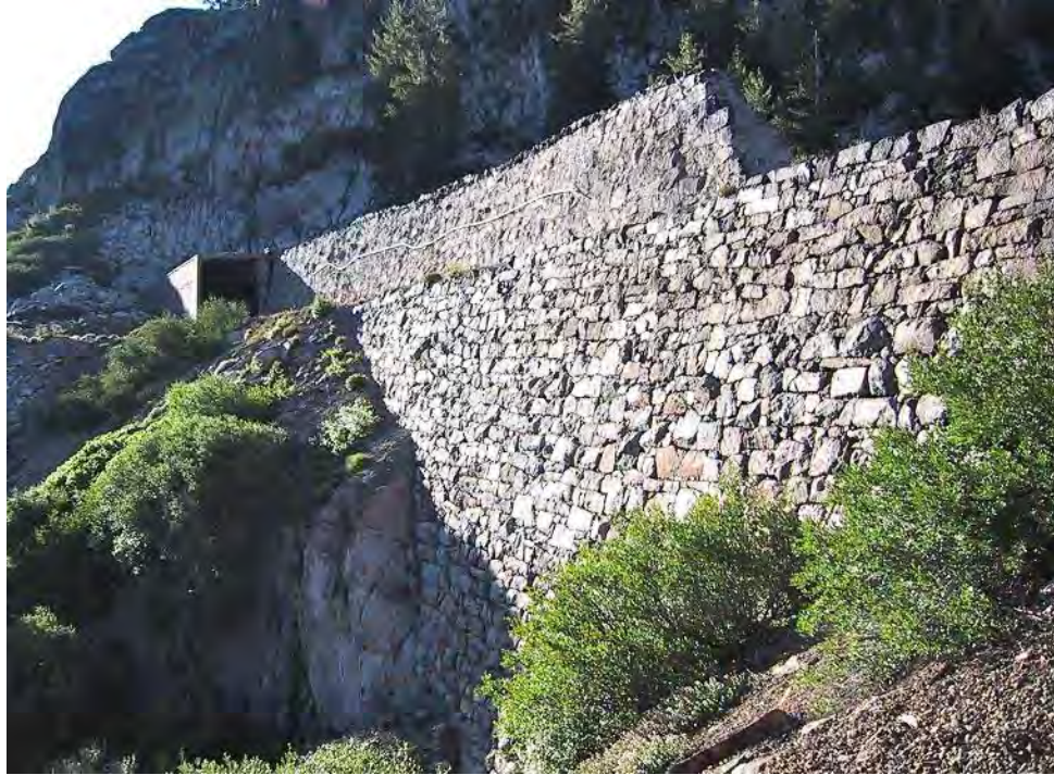
“China Wall,” constructed by Chinese laborers in 1869 to carry the Central Pacific Railway across Donner Pass, CA, 2004 (Arthur Gibbs Sylvester)
