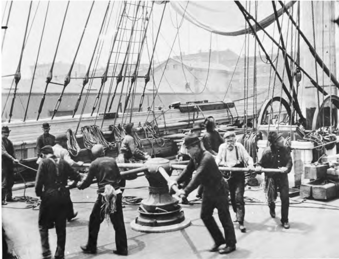
Crewmen turning a capstan on deck at South St., New York, NY, 1904 (San Francisco Maritime National Historical Park)
