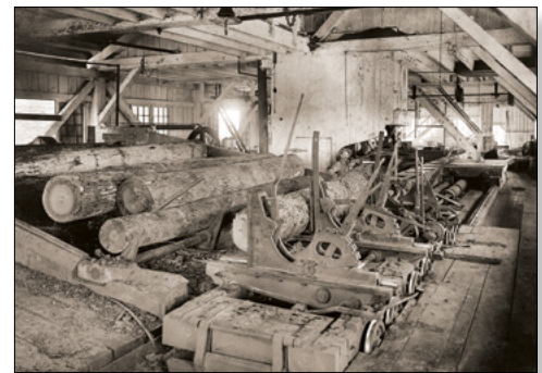
The mill carriage moves back and forth to carry logs to the band saw to be cut into lumber. A worker rides the carriage to move the log into position for cutting. The sawyer sitting near the large saw signals the settings that will determine the size of boards to be cut. (Photo from The History Center’s online collections [www.thehistorycenteronline.com])
