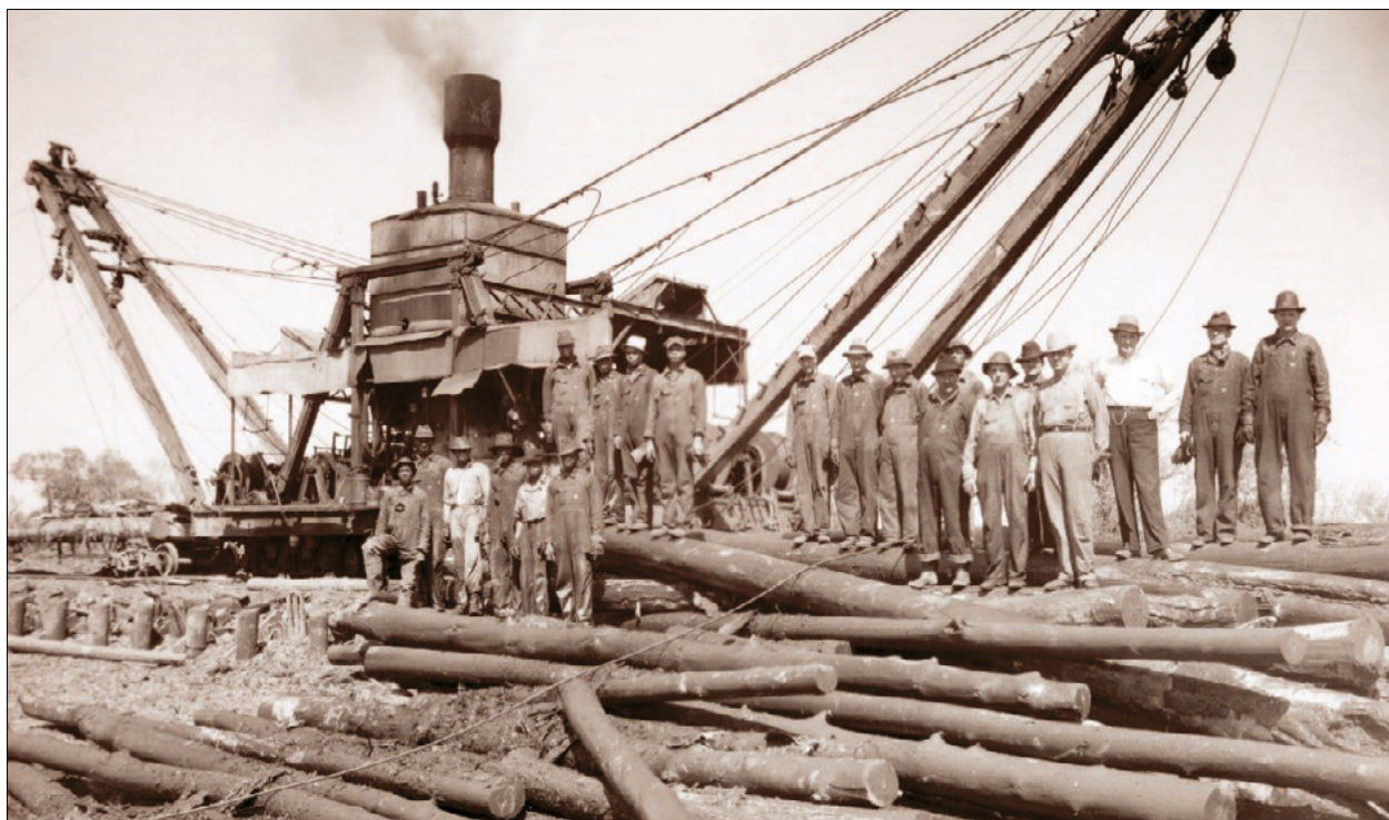
A Great Southern Lumber Company Clyde skidder with employees needed to operate the skidder and man the cables that pulled logs to the rail track for loading on log cars. These skidders could pull logs from 40 acres at one setting on the track. (Photo from Louisiana State University Archives
