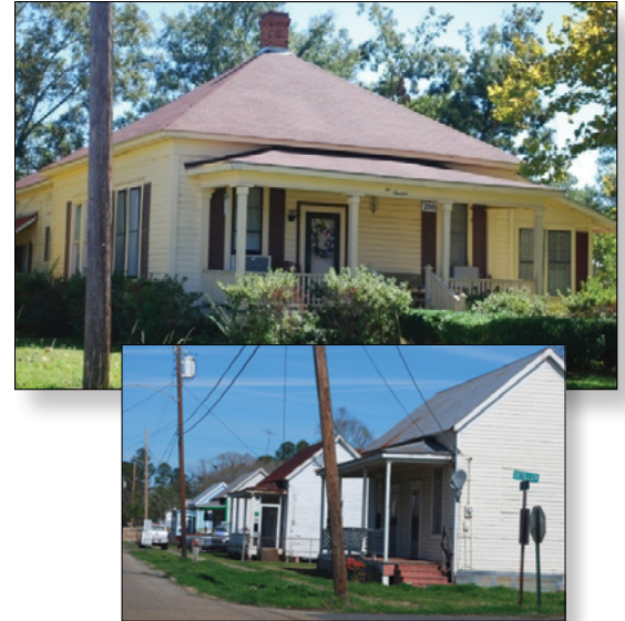
Recent photos of a pyramidal roof-style sawmill town house in Elizabeth (TOP) and log pen-style houses (BOTTOM) in Litcher, LA. Many of the early 20th century sawmill houses are still in use today, some left in place and others moved to different locations (Fricker [N.d.]).
