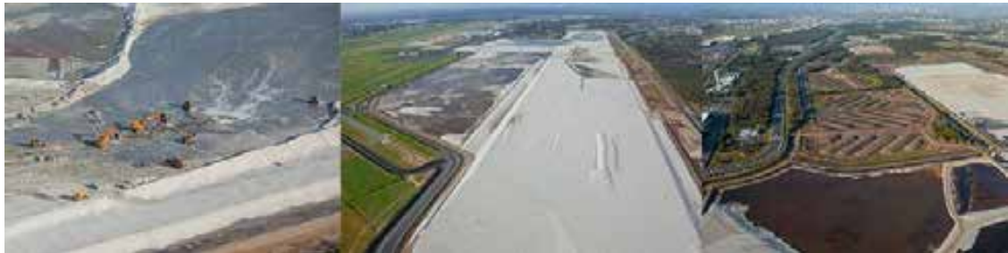
Figure 6. New Parallel Runway Project (3).
