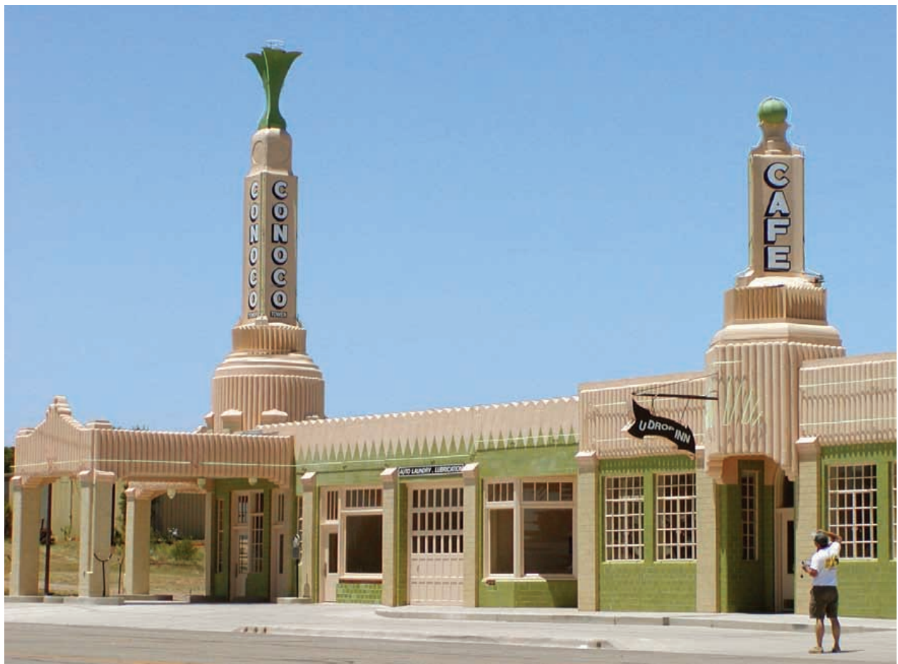
The Conoco Tower Station today.
