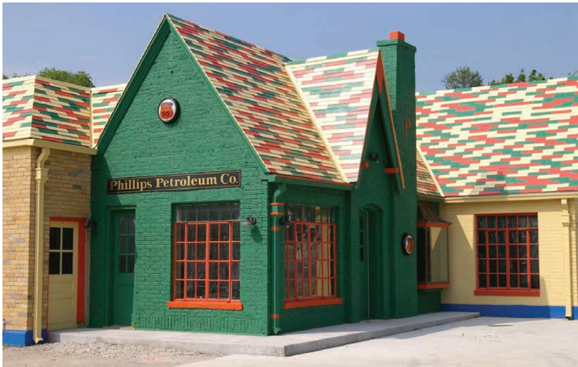
The Carr Service Station in Cuba has been fully restored to its original appearance, down to the original Phillips 66 trademark green and orange paint scheme.
