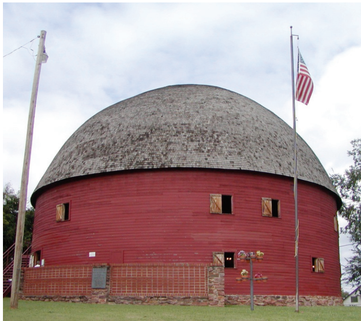
The Round Barn of Arcadia, Oklahoma, fully restored.
