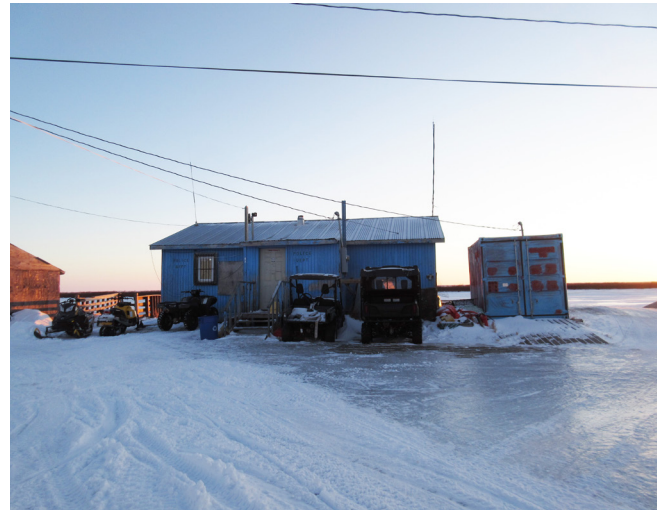
The police station in Atmautluak contains both an office and a jail cell.
