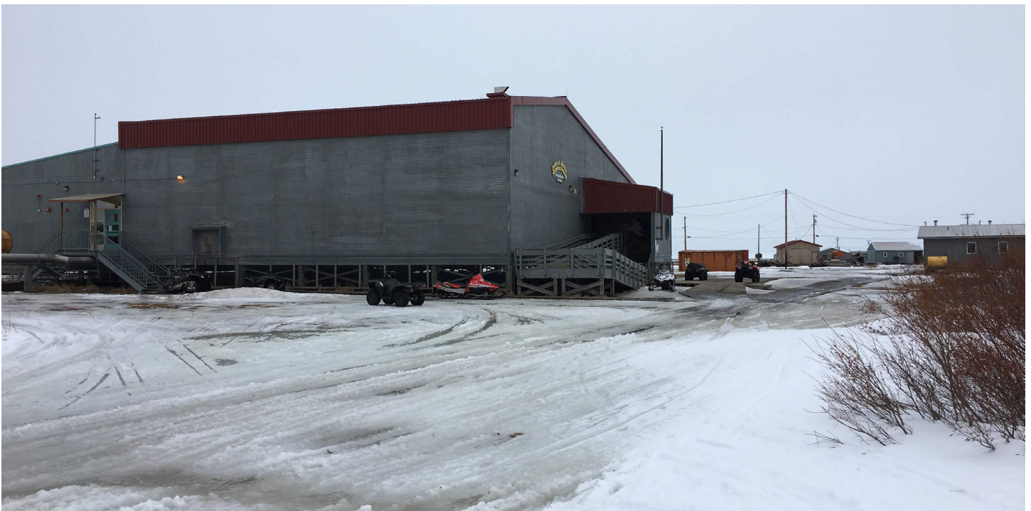
The school is a central building in Atmautluak. Not only does it host classes for all levels of students, it also serves as lodging for out-of-town visitors, and a gathering place for basketball games and sports tournaments.
