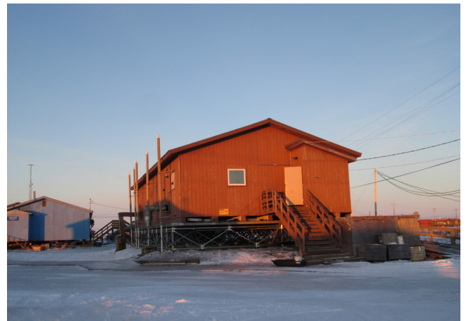
Waste heat from the power plant is utilized by numerous public buildings in the community, including the washeteria.
