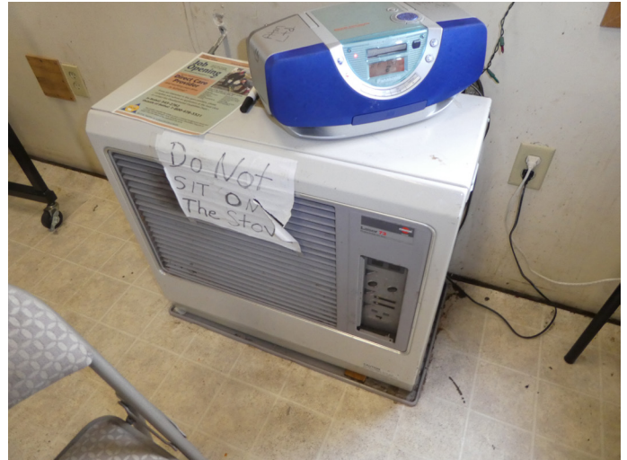
Check on the Toyotomi stoves periodically to ensure that the programmable thermostat is set to reduce the temperature at night.
