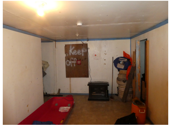
The Toyotomi stove in the police station should be checked on periodically to ensure that the programmable thermostat is set.
