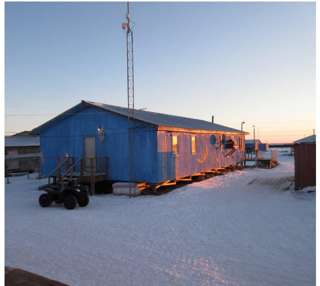
The gaming office's bingo hall takes up half of a repurposed building that sees great changes in occupant load based over the course of a typical week. The other half of the building is taken up by the post office.
