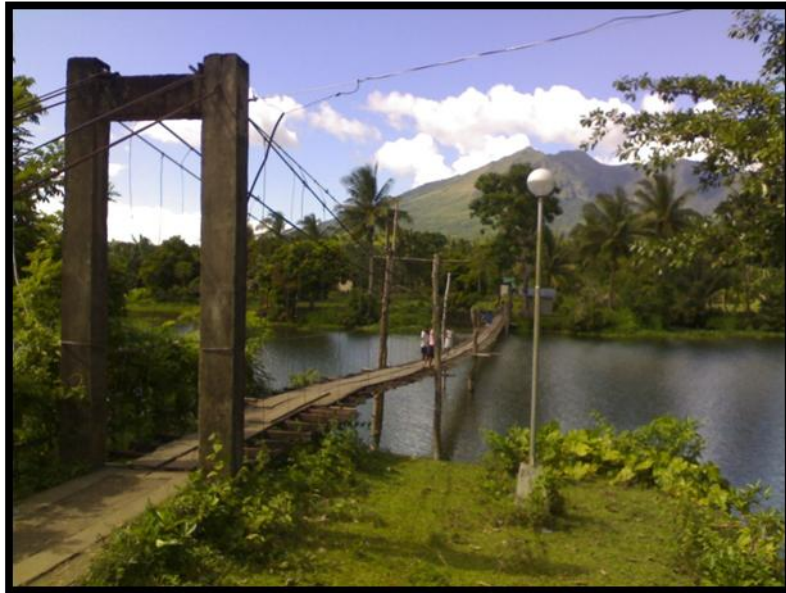
Figure 33 Hanging bridge connecting San Ramon to the main access road.
