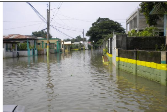
Bgy. Paralaya in Candaba still flooded as of 1300H, 29 June. Candaba water level station reading at about that same time was at 5.95 meters.
