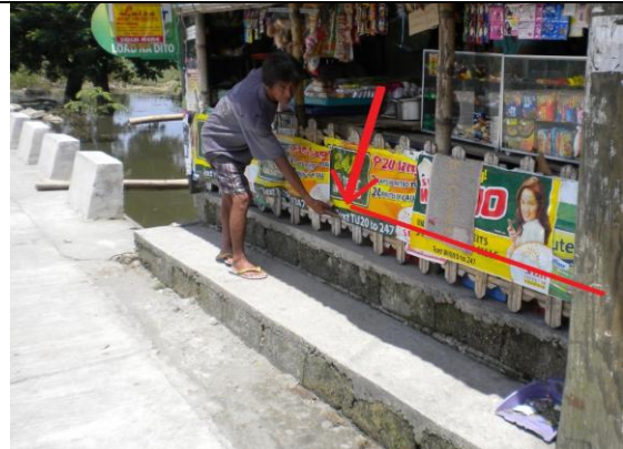
Flood depth of more than 0.5 meters from natural road level along the La Paz-Zaragoza Hi-way in Bgy. San Roque, La Paz, Tarlac.
