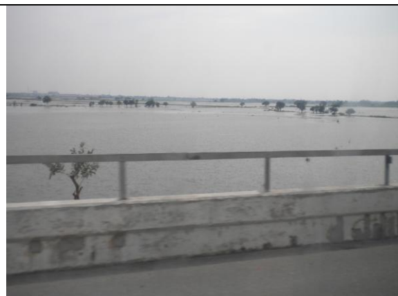
The lower Candaba swamp area as seen from the North Luzon Expressway (NLEX) viaduct. (29 June, 1500H)
