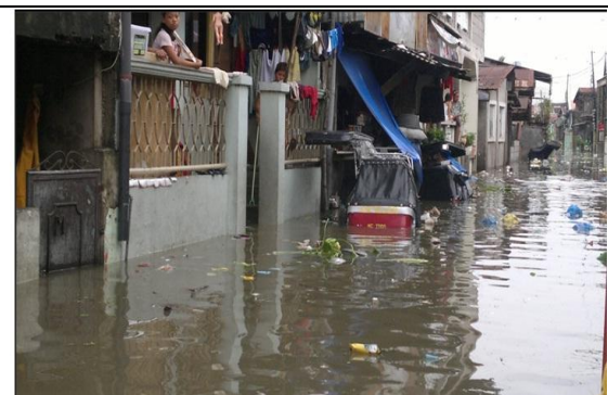
Flood situation of the interior roads of Bgy. Bancal, town of Guagua in Pampanga on June 25, 2011.
