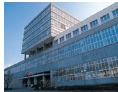
Operation building Otelfingen
