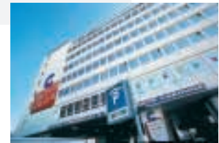
Carouge shopping center and offices
