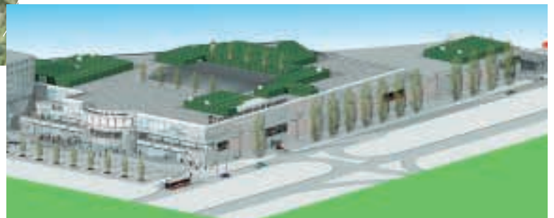
La Praille shopping center (under construction)
