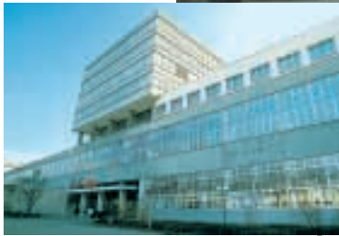
Office block and distribution center
