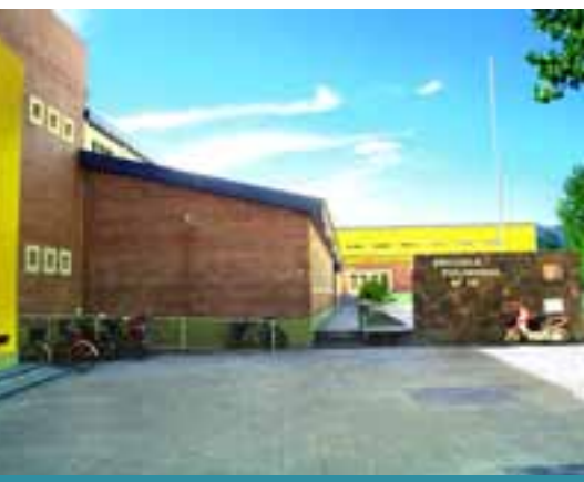
Construction of a technical secondary school in Belén, with a capacity for 1,700 students.
