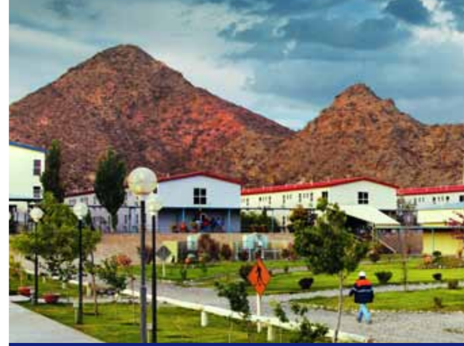
An overview of Bajo de la Alumbraera camp facility, including 480 rooms and recreational areas.
