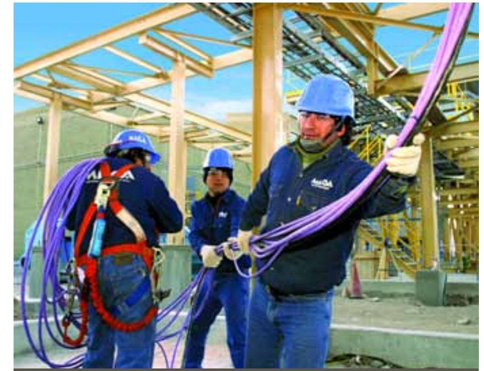
MEGA operators laying cables at our molybdenum plant.
