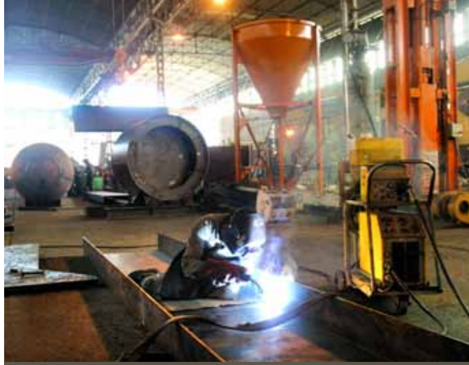
Repair of a Bucyrus shovel bucket at Di Bacco repair shop.
