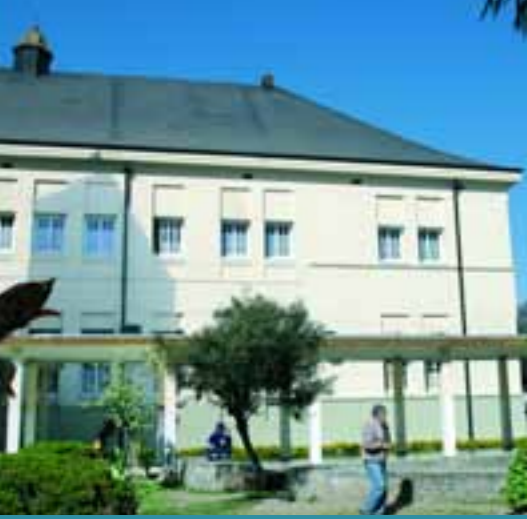
Remodelation of consulting rooms and hospitalisation area in the Obarrio Mental Health Hospital in Tucumán.
