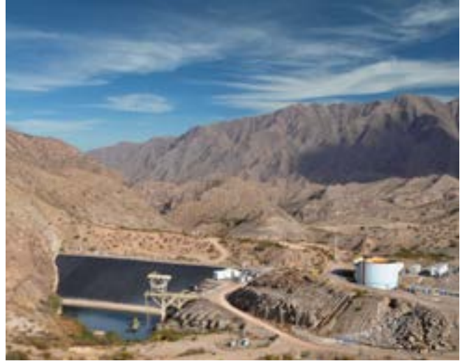
Reclaimed water collection pond.
