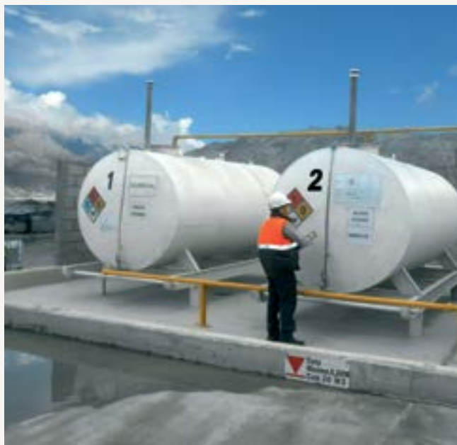
Hazardous waste (oil, grease, hydrocarbon-stained cloths) is stored at the site to be later transported and disposed by authorised companies.
