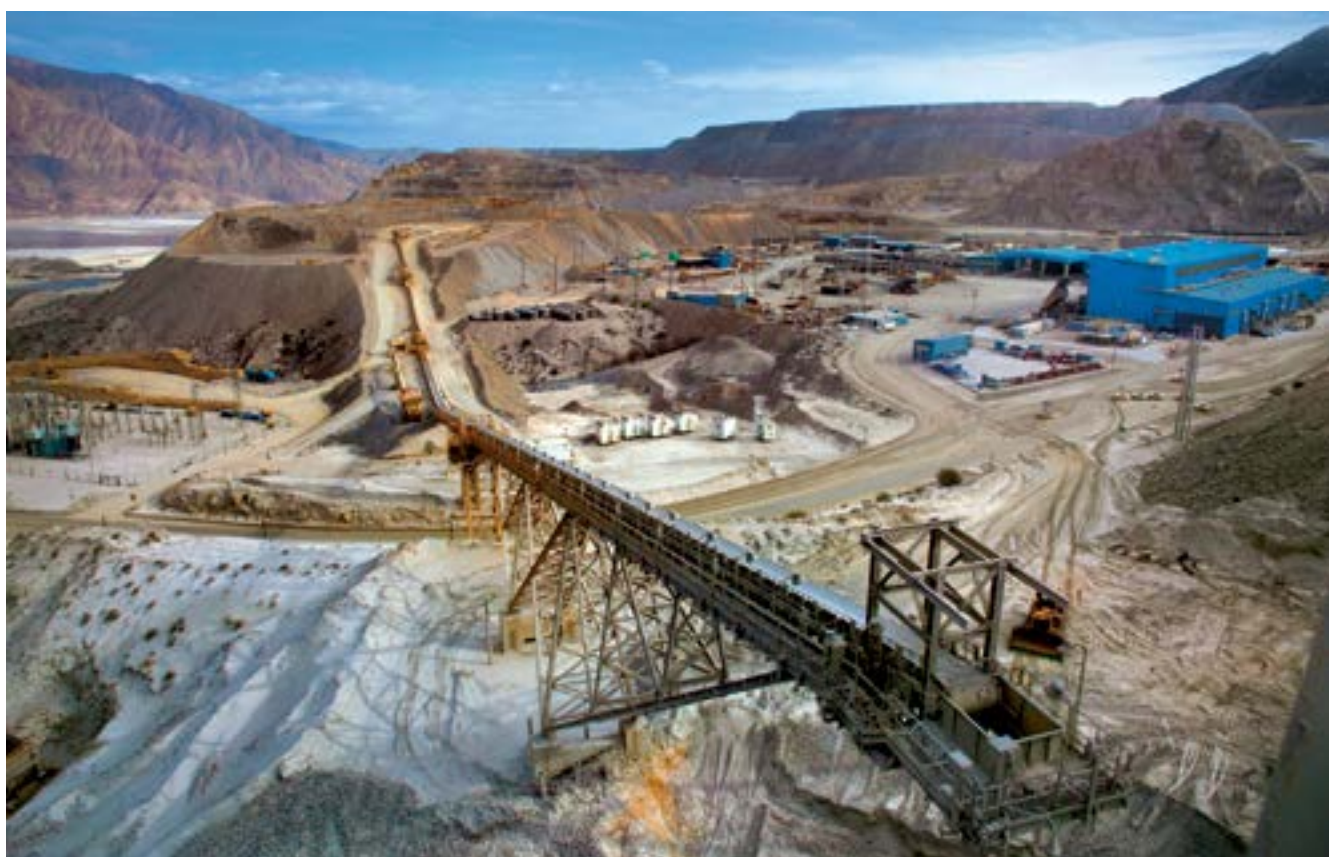
Overview of the feed circuit at the grinding plant.
