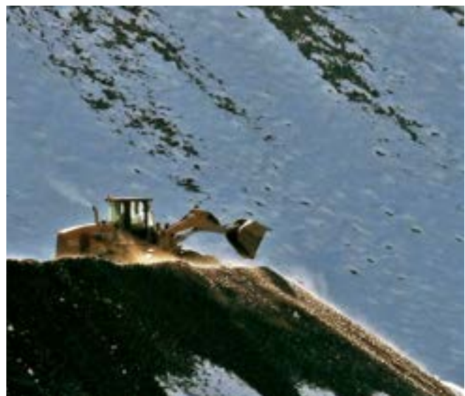
Road maintenance by loader in a snow-covered area.
