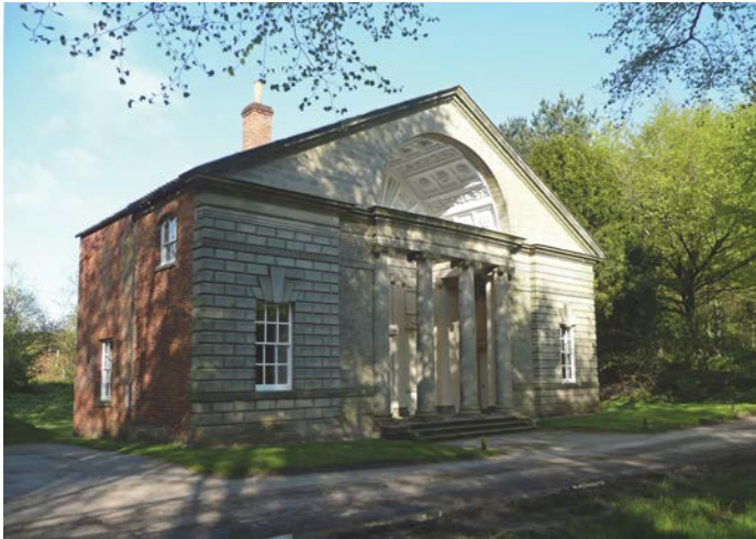
Restored Ingestre Pavilion
