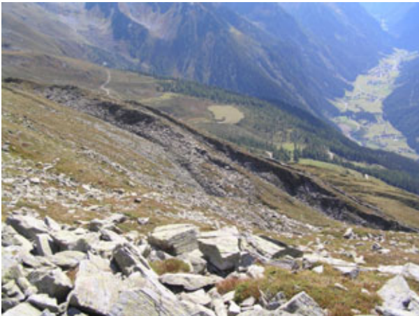
Figure 3 – Extensional cracks and scarps facing uphill.
