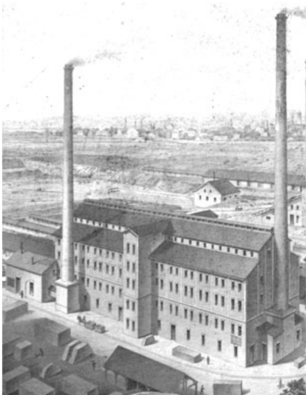
Figure 5 – The brick factory Jungmeier in the southern part of Straubing showing the extensive brickearth pits in the left background.
