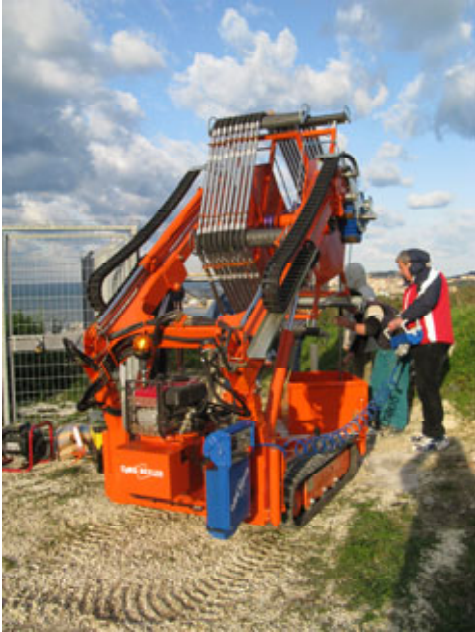
Figure 3 - DMS installation in place
