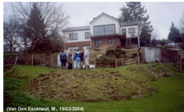
Figure 1 –Example of a landslide causing significant damage to a private property
