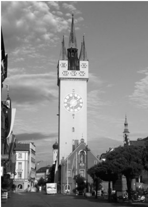
Figure 1 – The Gothic city tower of Straubing, standing on a Pleistocene terrace is a typical building with a combined brick and natural stone construction.
