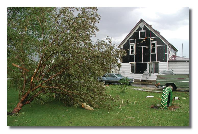
Pieces of lumber, siding and materials from garages, homes and businesses were projected into homes, cars and other objects in Bradgate. The small 'missiles' as the National Weather Service calls them, accumulate speed and embed themselves into any object they come in contact with. The piece of roof shown below is similar to one that was also thrust into the Edler home, pictured above.
