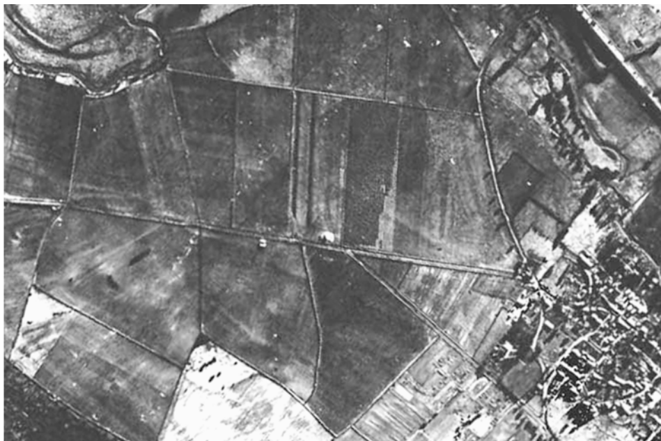
Fig. 16. Enclosures by local agreement often left existing road systems intact, whereas parliamentary enclosures gave power to change them. These two 1947 air photographs illustrate how these two processes can create differences in the landscape. Both Ashwell and Teigh were enclosed by local agreement in the seventeenth / early eighteenth century, and the upper photograph shows the road between them continuing to meander around old open field boundaries. In contrast, the lower photograph of Barrowden shows the new straight roads created by surveyors during its enclosure in 1882 (English Heritage (NMR) RAF Photography)
