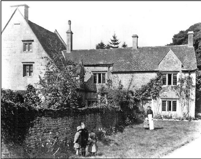
A 1913 photograph of The Old Rectory when it was two dwellings. (Jack Hart Collection)
