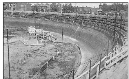
Luna Park Motordrome in Cleveland, Ohio (top) and the St. Louis Motordrome in Missouri (bottom). Some of the motordromes had turns banked at 62 degrees!
