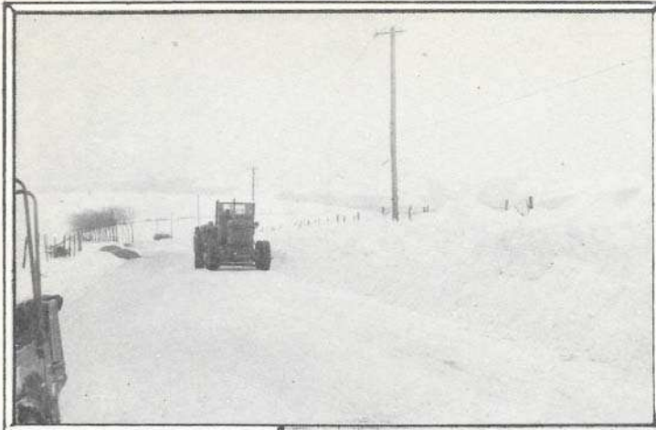
FIG. 2 Gallion Grader clearing snow from ARSDORF- BOULAIDE Road
