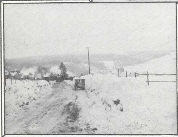
FIG. 3 R-4 Caterpillar Tractor clearing snow on ARSDORF- BOULAIDE Road
