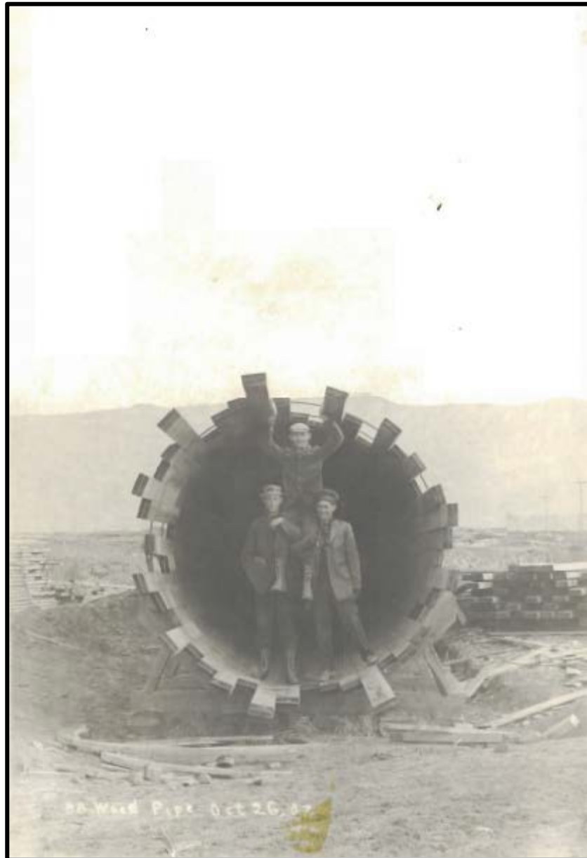
Figure 4.8 Men standing inside wood stave, October 26, 1907 (Courtesy PacifiCorp).
