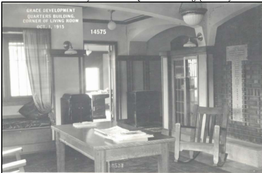
Figure 5.10 Interior view of UP &L Quarters Building. (Courtesy PacifiCorp).
