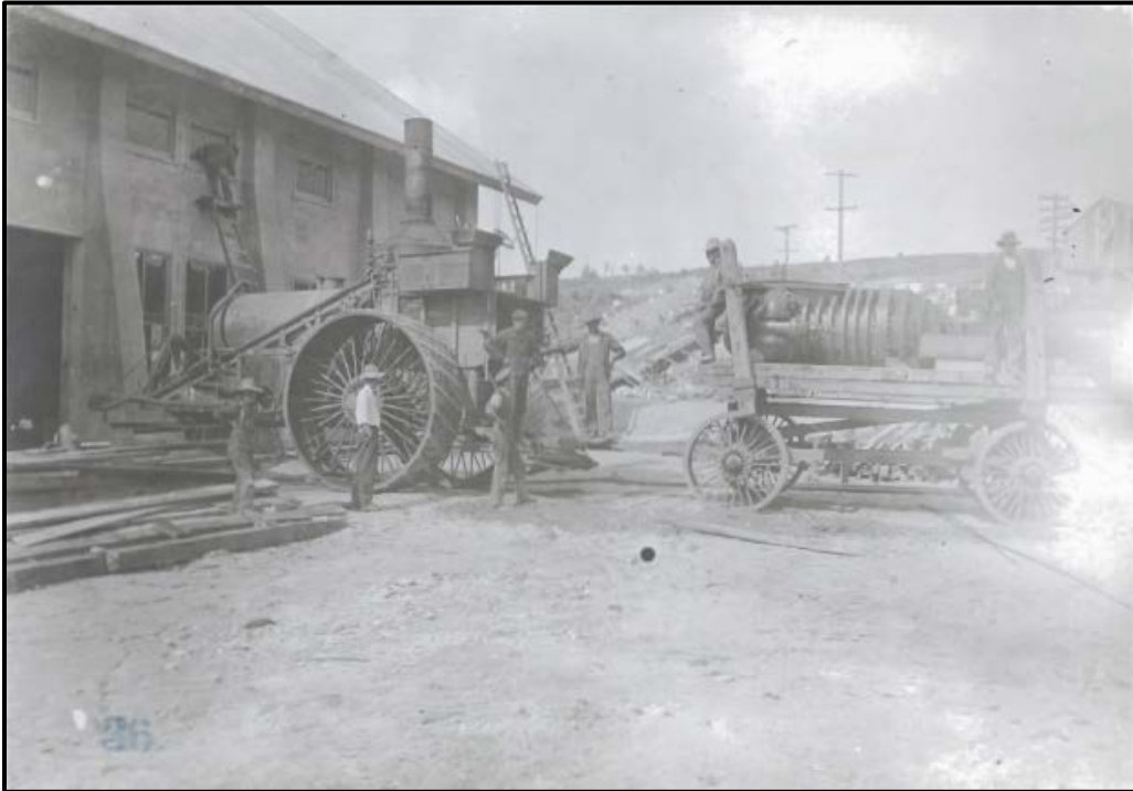
Figure 4.11 Construction workers completing detail work on the powerhouse. 1907. (Courtesy PacifiCorp).
