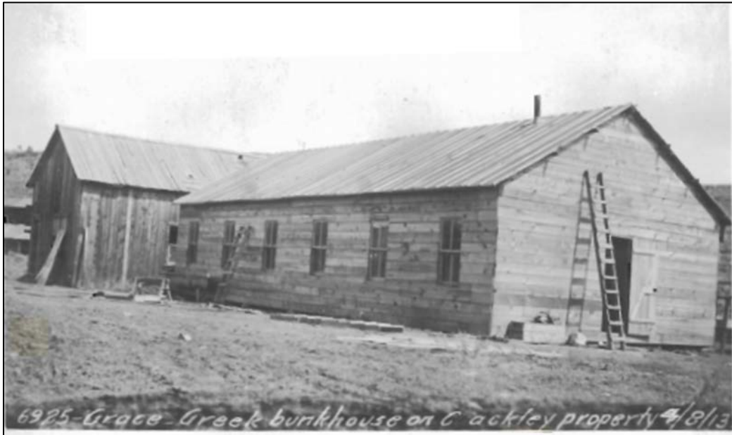
Figure 5.3 Approximately 100 men were divided among the construction camps. (Courtesy PacifiCorp).
