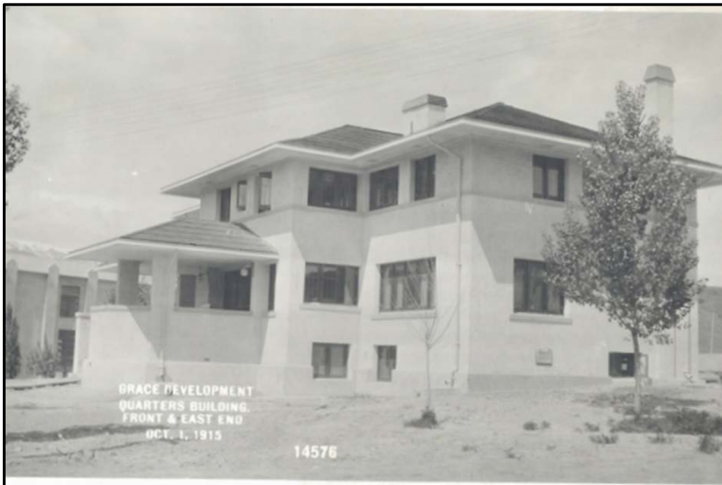
Figure 5.8 Shown above is the new Quarters Building constructed by UP&L in 1915. (Courtesy PacifiCorp).
