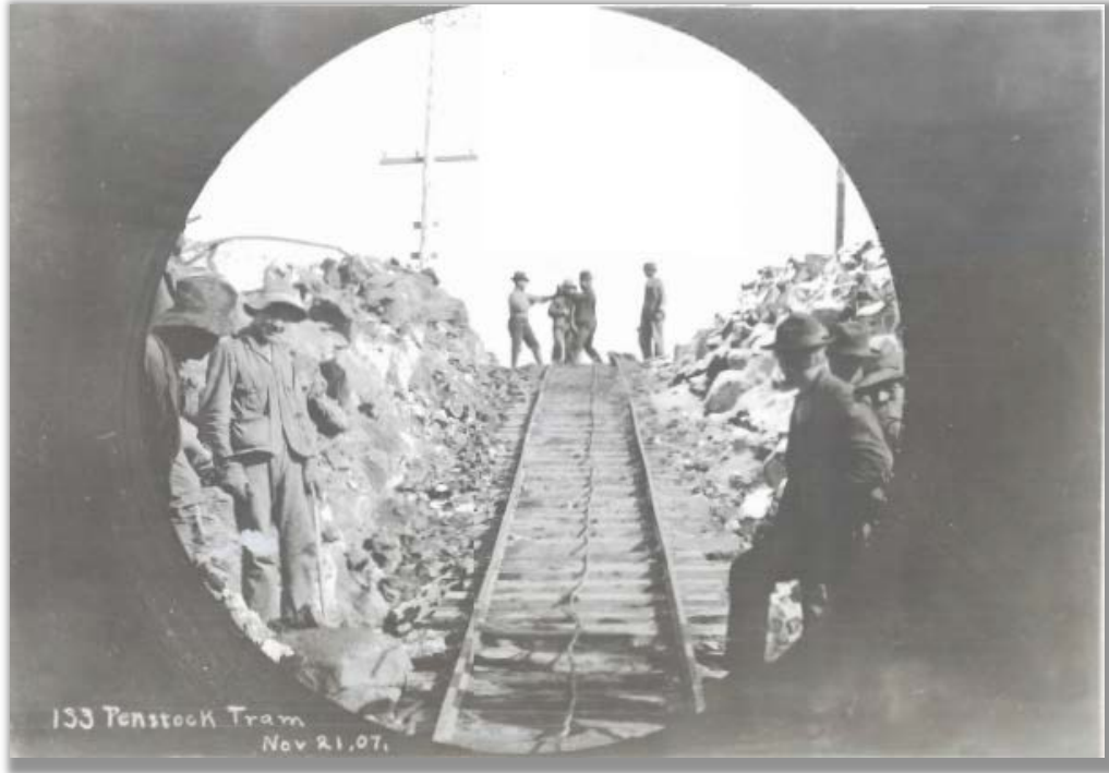
Figure 4.9 View of penstock tram from inside the eight-foot diameter steel pipe, November 1907. (Courtesy PacifiCorp).
