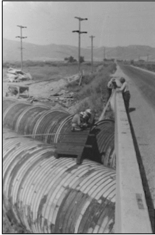
Figure 5.15 Few historic images of the Turner Road Penstock Bridge exist. This 1952 construction photo shows men standing on the bridge over the flowlines. (Courtesy PacifiCorp).
