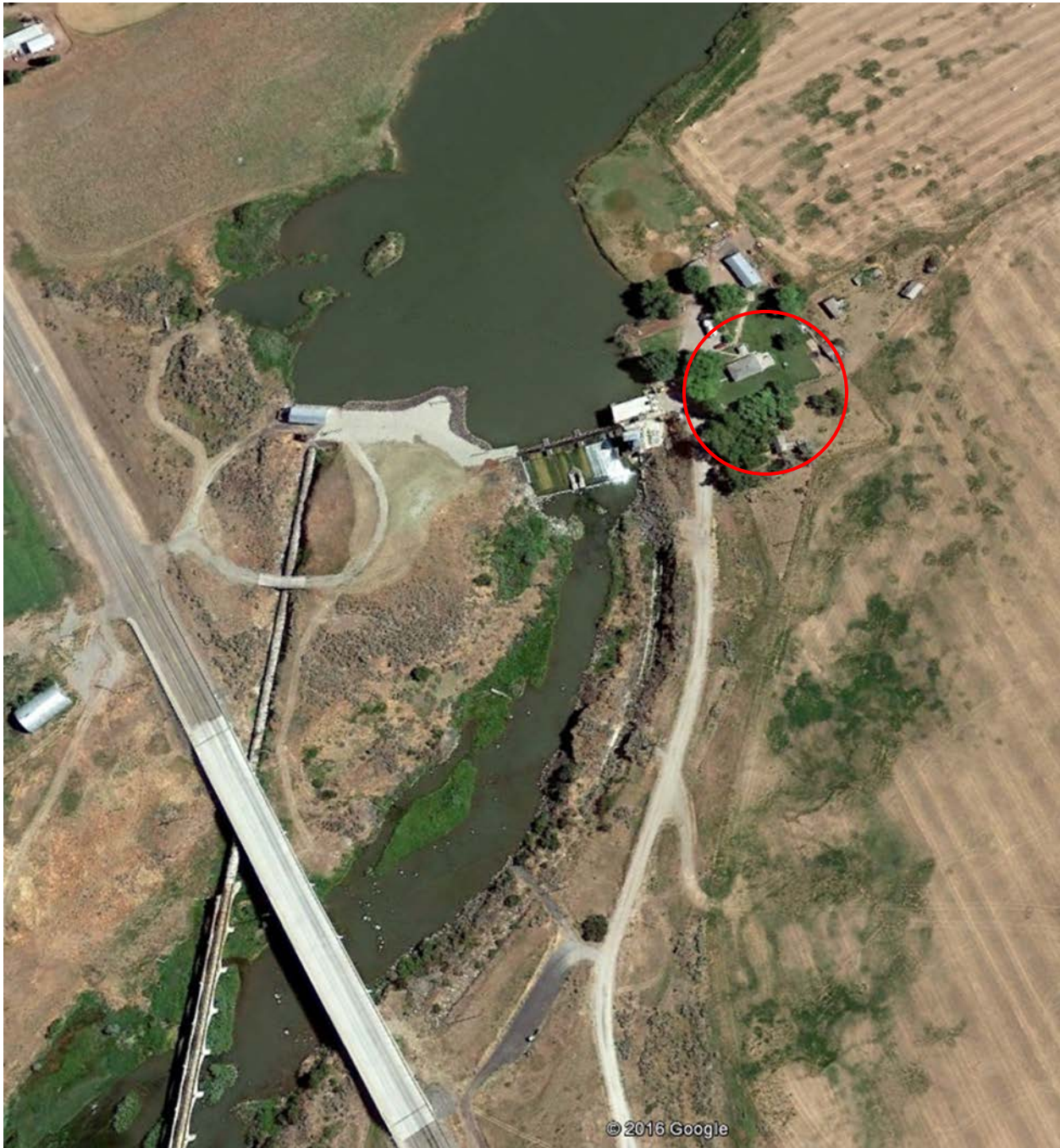
Figure 5.14 2016 Google image showing layout of Grace Diversion Dam and Dam Tender's Residence. Residence shown in red circle.
