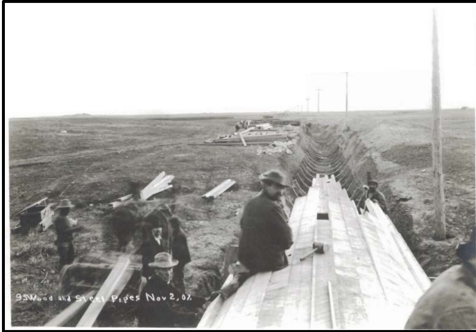
Figure 4.6 Construction crew building four-mile long wood flowline and steel penstock, . November 2, 1907. (Courtesy PacifiCorp).
