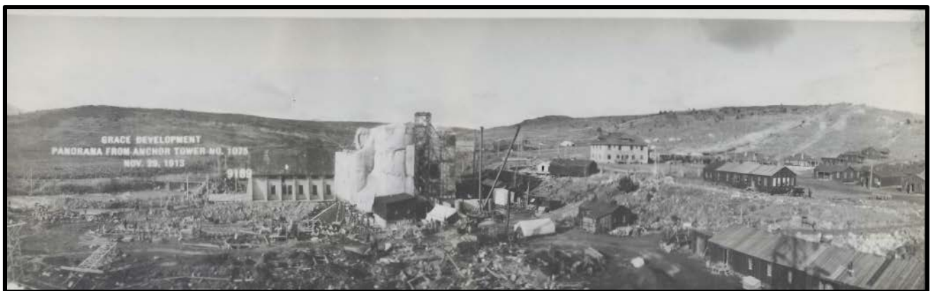
Figure 5.16 View of Grace Development and construction of new dam. (Courtesy PacifiCorp).
