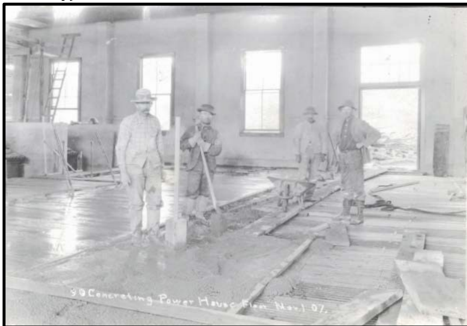
Figure 4.12 Men spreading concrete for powerhouse floor. November 1907. (Courtesy PacifiCorp).
