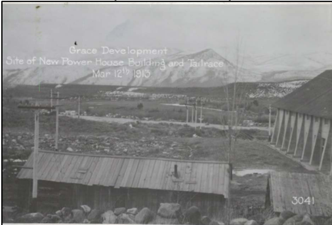
Figure 5.5 The site of the new power house shown adjacent to the 1908 one. (Courtesy PacifiCorp).
