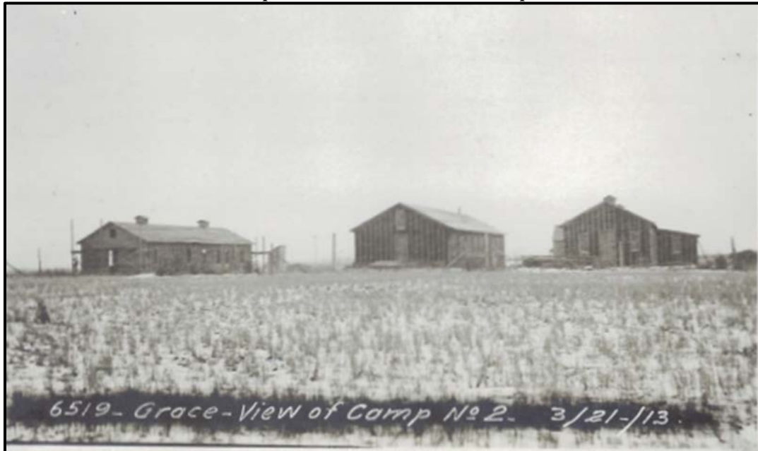
Figure 5.1 Construction camps were built near the dam and power plant. (Courtesy PacifiCorp).
