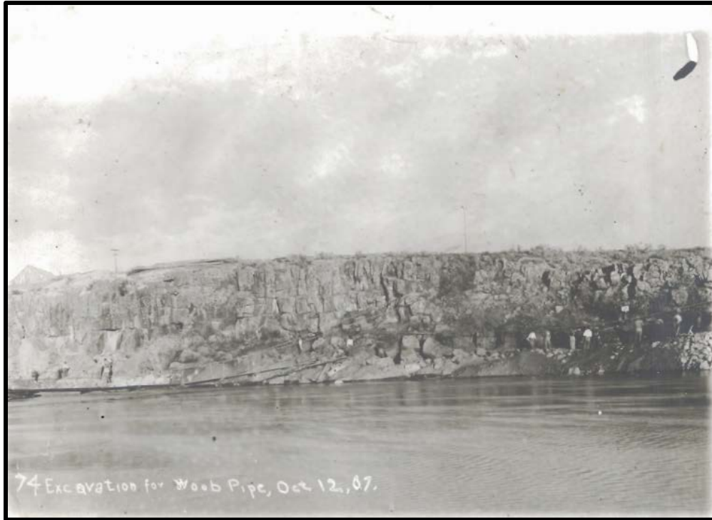
Figure 4.3 Excavation for flowline October 12, 1907. (Courtesy PacifiCorp).
