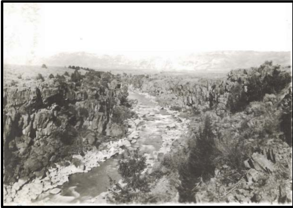
Figure 4.2 View of Bear River Canyon from construction photos of Grace Dam, 1907. (Courtesy PacifiCorp).
