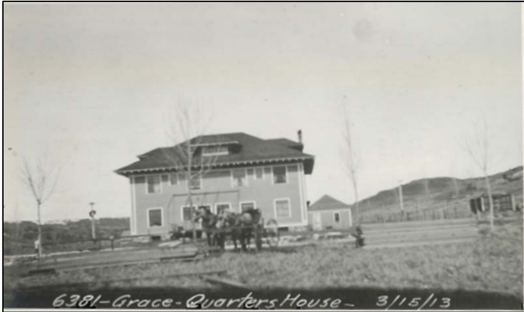
Figure 5.7 L.L. Nunn built quarters for the construction crew in 1908. The building burned down in 1914. (Courtesy PacifiCorp).
