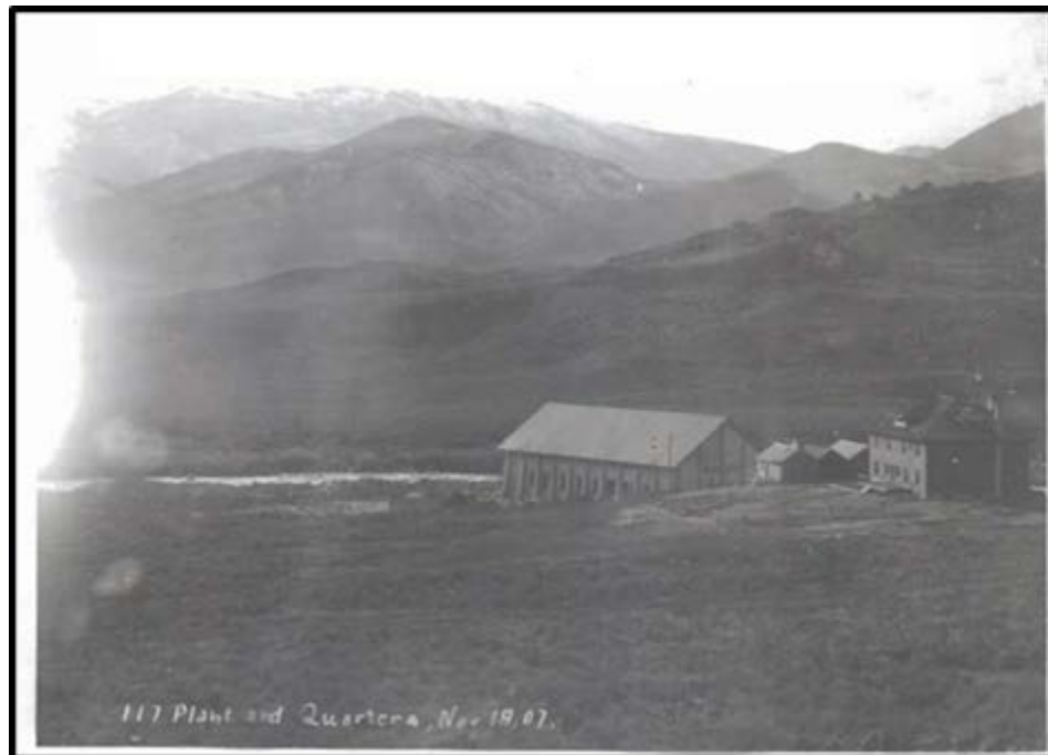
Figure 4.14 The finished Power Plant included the dam, flowline, and surge tank. Staff quarters are shown at right in the photo. This building burned down in 1914. (Courtesy PacifiCorp).
