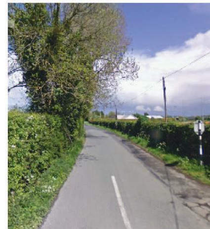
New and widened footpaths
