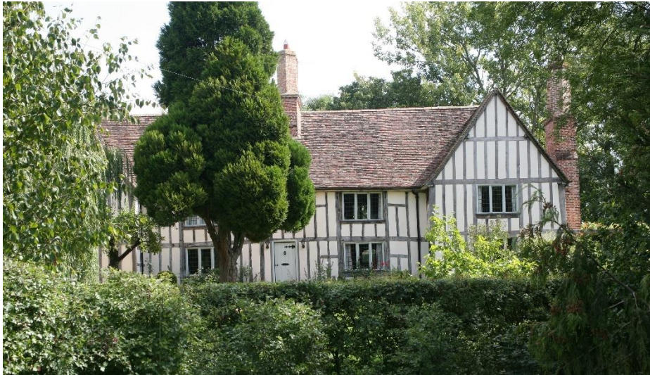
Dobbins Cottage (also known as Town Farm House) Grade II
