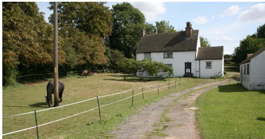
The Poplars (originally known as Hospital Farm House) Grade II
