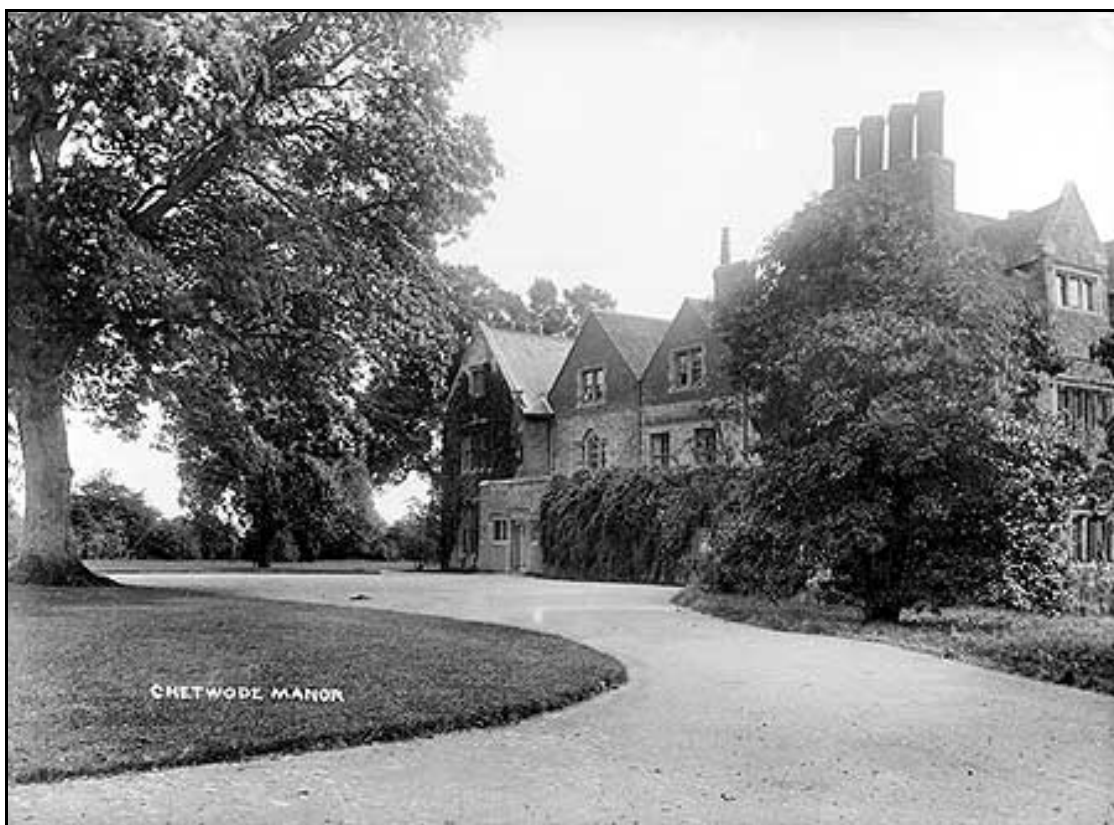
North front and forecourt, c.1896-1920 (Historic England BB98/01950).
