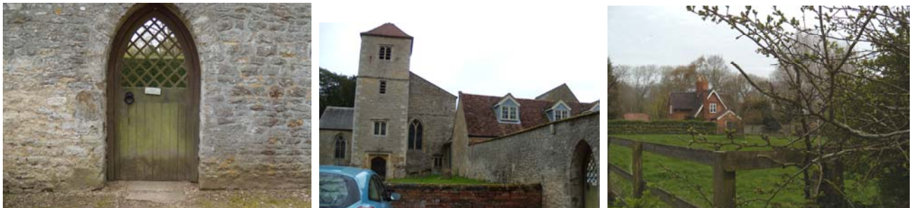
Forecourt gateway to church (left); church, west front (centre); kitchen garden and gardener's cottage (right).
