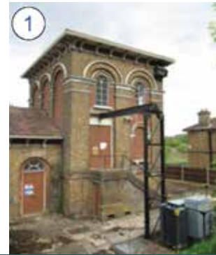
Amwell Marsh Pumping Station
