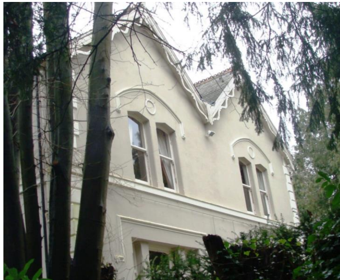
Picture 14. Good quality window surround, quoin and barge board detailing worthy of retention and protection.
