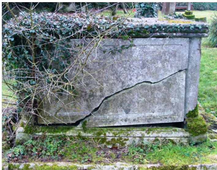
Pictures 20-22. Upper - General view of historic churchyard; lower two historic chest tombs in urgent need of renovation/repair/removal of ivy. The potential of seeking grant assistance is worthy of consideration.
