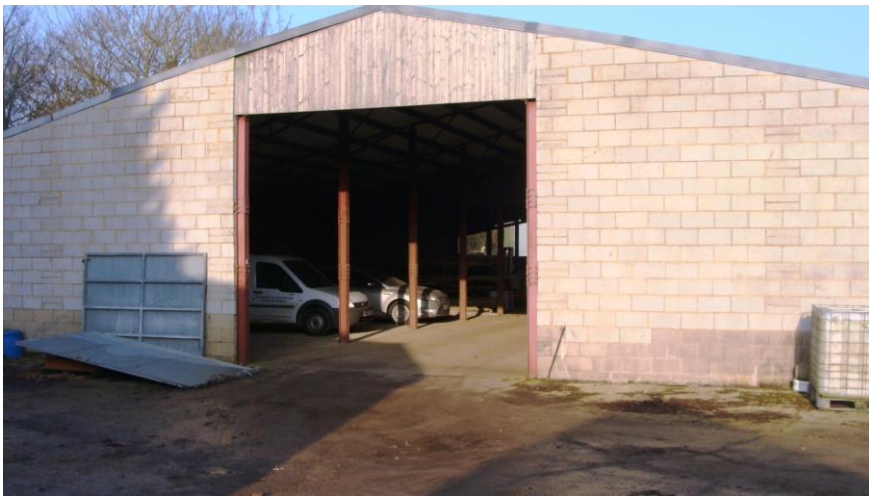
Pictures 34-35. Mid and later 20th century utilitarian buildings associated with Aspenden Hall proposed to be removed from the conservation area.
