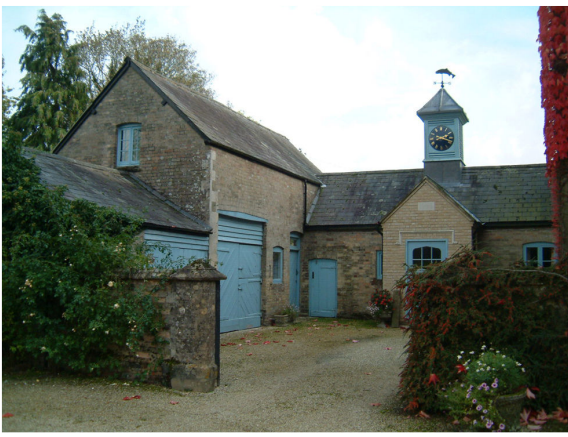
The Old Rectory. Slate roofs on the coach house
