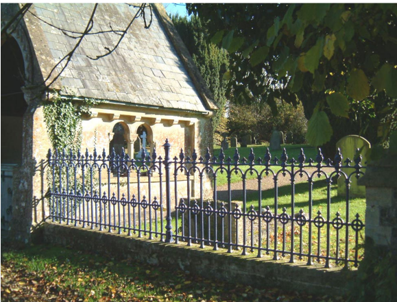
St Nicholas Church. A slate roof on the lych gate limestone walls and fine quality iron railings .
