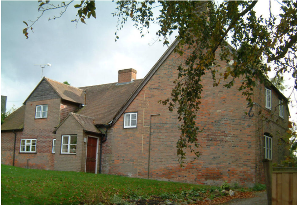
The plain character of 20 th century brick and tile of the roadside aspect of East Grafton Farmhouse
