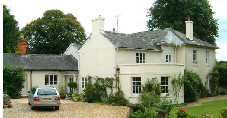
Green Hall. The grounds of lawns, shrubs and trees compliment the house and are an asset to the Conservation Area
