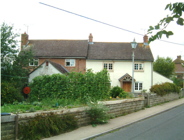
Wilton Road. Cottages No. 230 and No 229. The roadside concrete wall, pavement and low kerb
