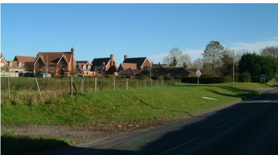
Grafton Place. Exposed large scale houses of a development in an open green field site on the edge of the village. The excessively wide visibility splays detract from the vulnerable rural character of the Conservation Area. Some tree planting on the western edge of the housing and hedging along the roadside would soften the impact of this standard type of development.
