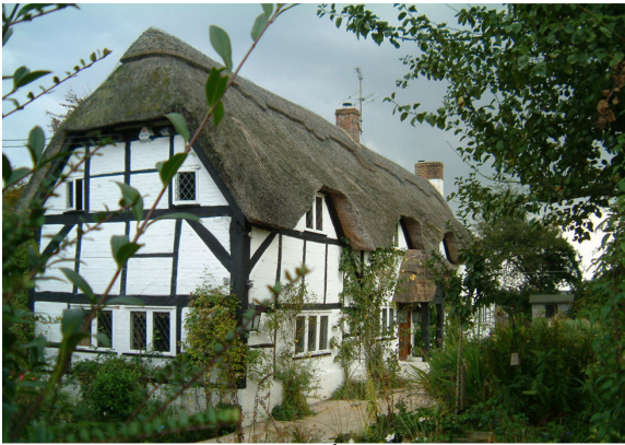
Timber framing of the 17 th century with both surviving wattle and brick nogging infill panels
