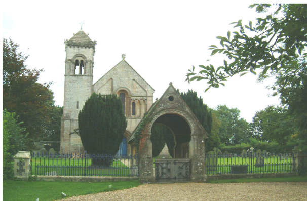
The lych gate and railings were erected soon after the Church of St Nicholas of 1845
