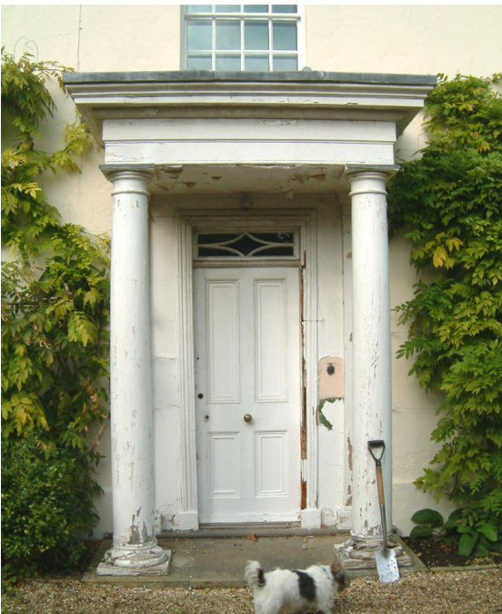
Green Hall. c1830 Stucco on brick with finely barred sash windows, panel door, over-light and timber entablature with columnar supports.
