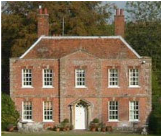
A plain clay tile roof with lead rolls over hips Red brick walls with stone dressings. Timber sash windows and a panel door with a fanlight
