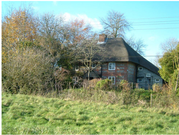
Flint Cottage looks out from among the trees
