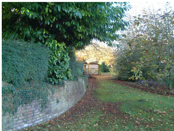
Tidcombe Manor. This curved retaining wall is a fine feature facing the lane on the north side of the house.
