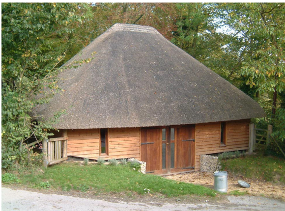
Flint Cottage. A reconstructed timber outbuilding with thatched roof and traditional weatherboard cladding.
