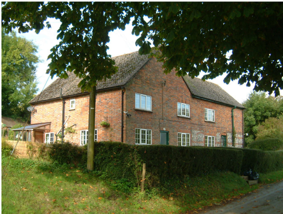
Cottages No.s 10 and 11 are pre 1880 but was largely rebuilt in 1950
