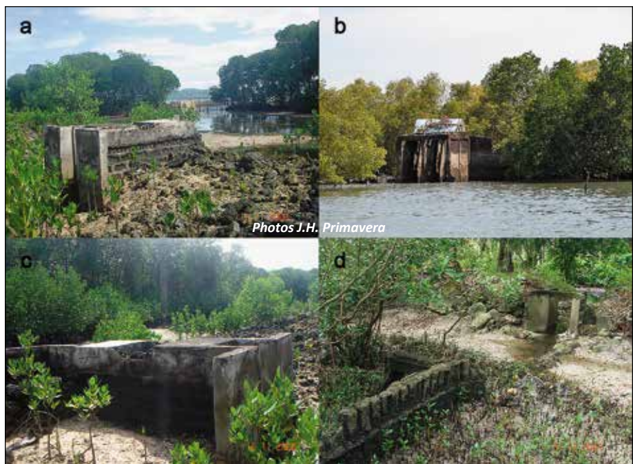
FIG. 9. Concrete gates are the only evidence that these sites in a, c) Calatagan, Batangas, b) Barotac Nuevo, Iloilo, and d) Tangalan, Aklan were once culture ponds. Natural regeneration back to mangroves takes 15-20 yr.
