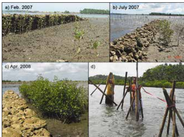
FIG. 32. Barriers made of a, b, c) rocks in Ermita, Dumangas, Iloilo (2007-2008), and d) bamboo in Balarig, Ivisan, Capiz (experimental) support mangrove growth by reducing wave energy and trapping sediment.
