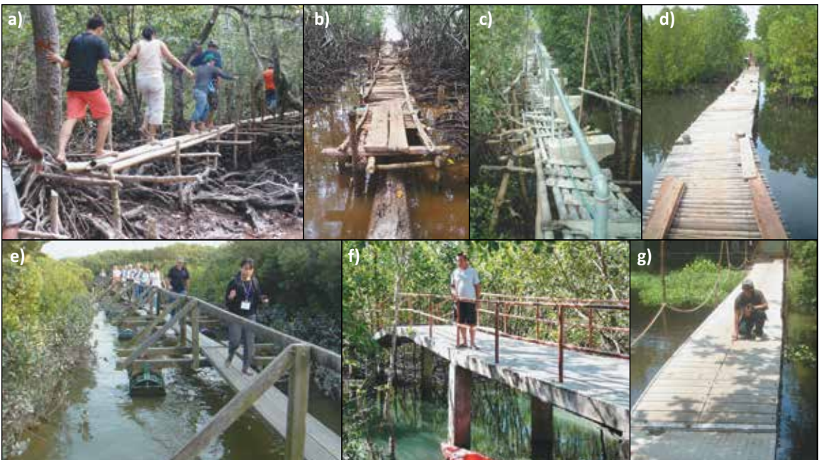
Fig. 8. Boardwalk types. a) Damaged bamboo, Masbate and b) wooden planks, Puerto Princesa; c) bamboo replaced by concrete, Badian, Cebu; d) wooden boardwalk without railing, Zamboanga City; e) floating boardwalk with railing, Mai Po, HK; f) concrete footwalk, Silonay, Mindoro Or.; and g) composite wood decking boardwalk, Sungei Buloh, Singapore. Photos by J.H. Primavera.
