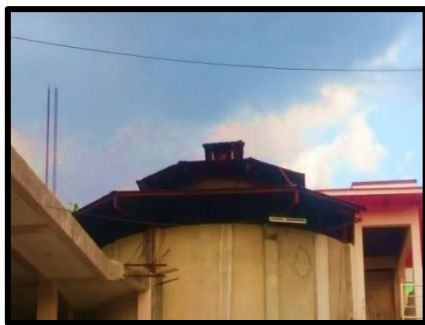
SIREN ALARM SYSTEM
