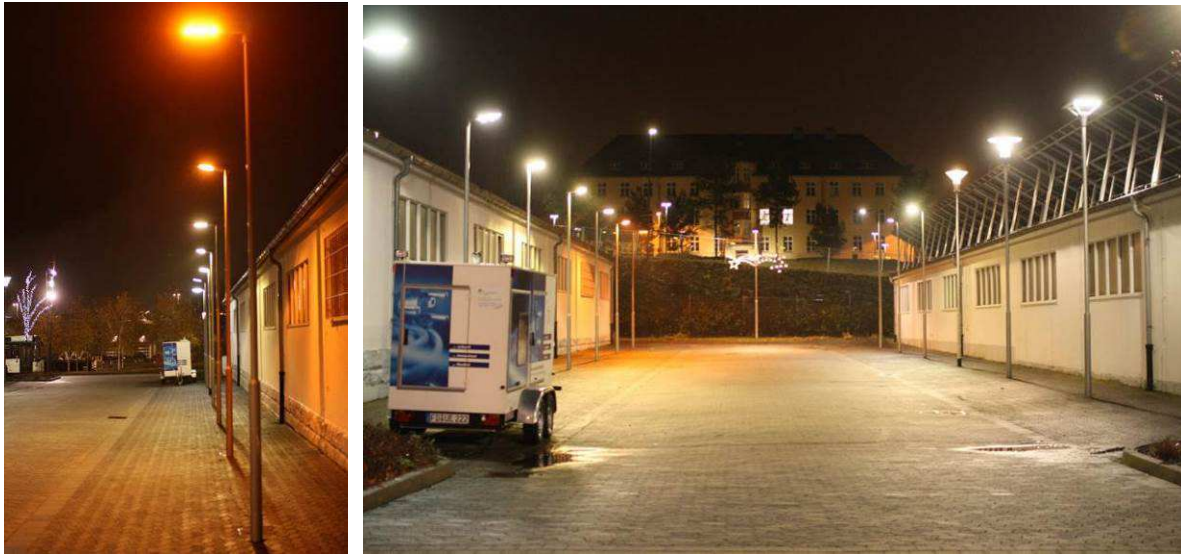
Fig. 9.19: The lighting test road of RhönEnergie in Fulda with PC-amber LED lighting
