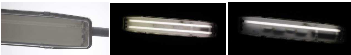
Fig. 9.18: Luminaires in Hilders are mostly equipped just with one fluorescent tube instead of two.
