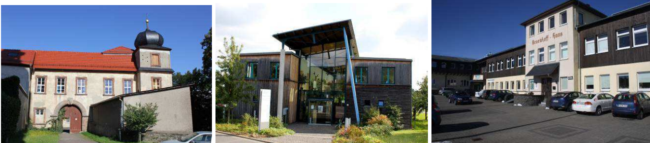
Fig. 5.9: The three Biosphere Reserve administrations in Zella (Thüringen), Oberelsbach (Bayern) and the Wasserkuppe (Hessen)
