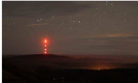
Fig. 7.13: TV tower Heidelstein.with security (air traffic) lighting.
