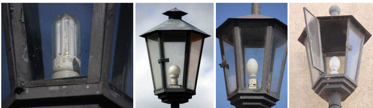
Fig. 9.15: The Fladungen luminaire was used with different kinds of lamps (left: 2 CFL with 16 W, then sodium high pressure with 68 W, and these were changed through the door (right))
