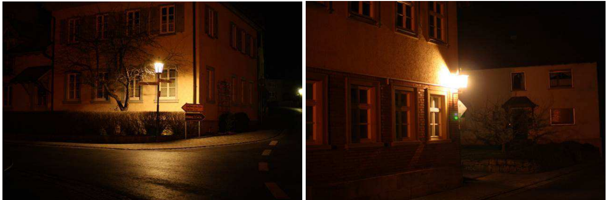
Fig. 9.9: Left: test retrofit installation with a LED module mounted in the roof of the lantern. Right: a conventional sodium high pressure lamp with high ULR.
