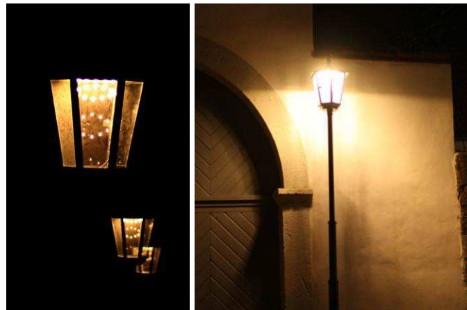
Fig. 9.17: With the renovation a LED board was installed in the roof of the luminaire. There is only little upward light and most of the light is emitted downwards.
