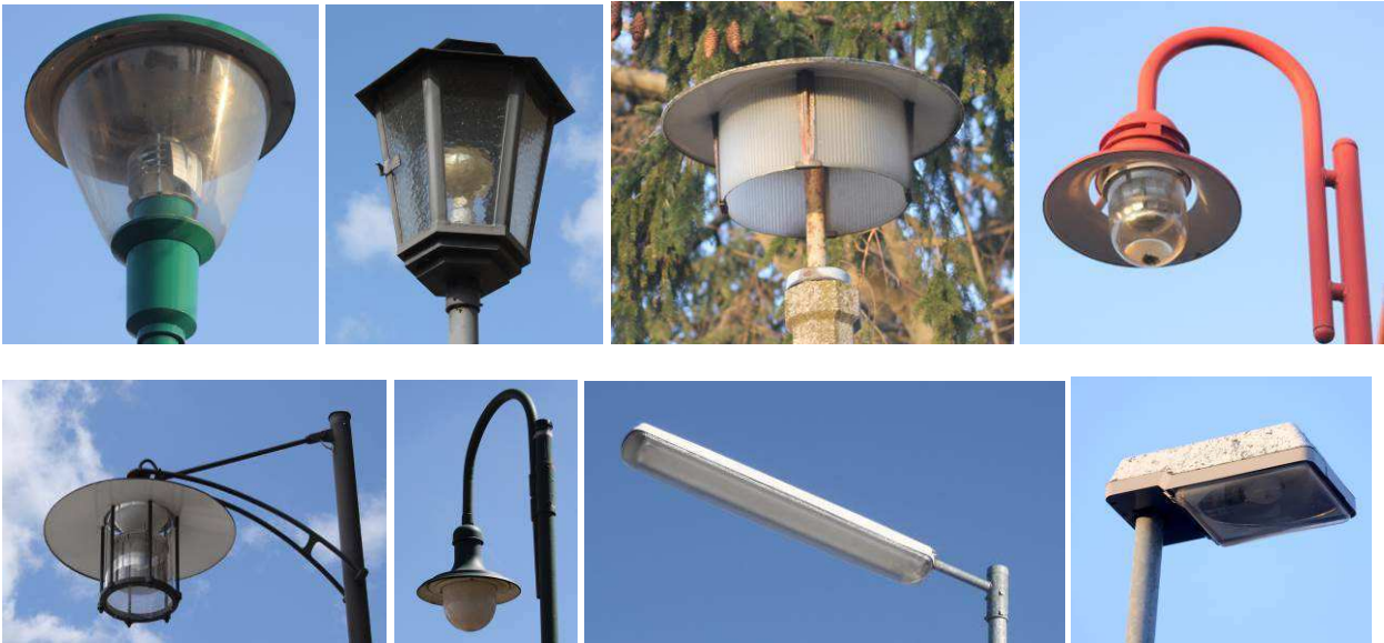
Fig. 7.21: Typical luminaires in the Rhön. The fixtures in the top row and the two at the bottom left have typically ULR = 10-25 %, the others have typically ULR = 5 and 2 %.
